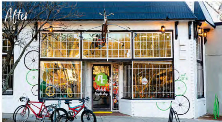
A/C Clutch Façade Renovation, Artist Partners: Rose Smith & Morgan Myles. Source: https://beltline.org/the-project/economic-development-commercial-real-estate/business-facade-partnership-grant-program/#past-projects
