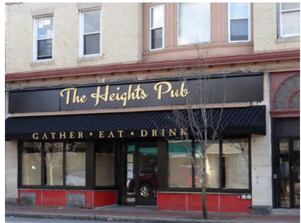
Heights Pub – After. Photo: FinePoint Associates
