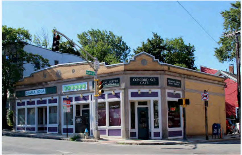
The owner of 290-294 Concord Street used SIP funds to update the building façade and make the entrances and display windows more inviting. Automatic door openers were also installed to make the stores more accessible. Source: City of Cambridge
