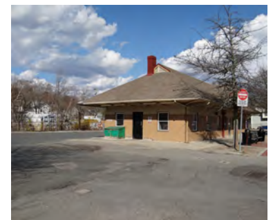
Under-utilized MBTA building and surrounding lot. Photo: FinePoint Associates
