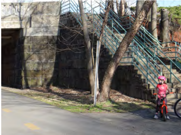
Bikeway stairway access to Park Ave. Photo: FinePoint Associates
