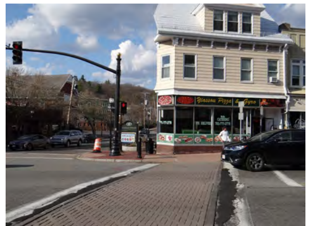
Crosswalk and curb extension on Mass Ave at Park Ave. Photo: FinePoint Associates
