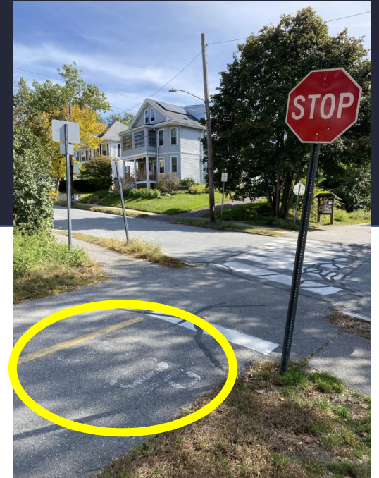
"STOP" marking is faded
