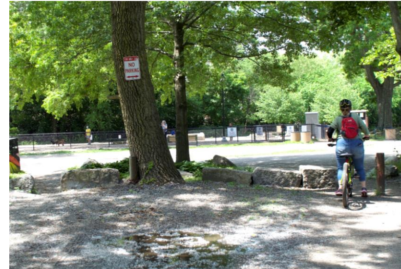
Drainage issues, surface material, and vertical elements inhibit ADA access
