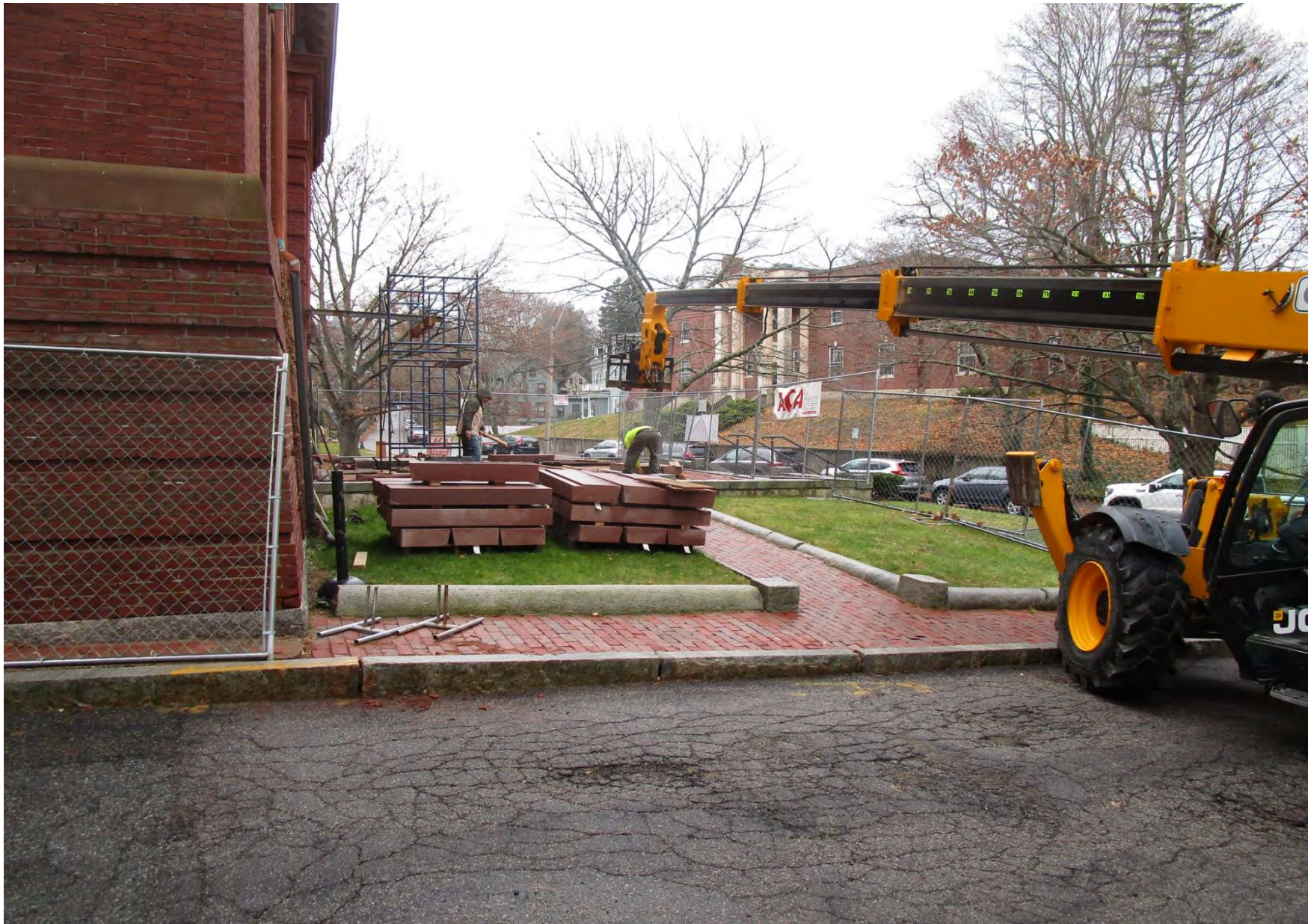
Installation of precast stone stairs
