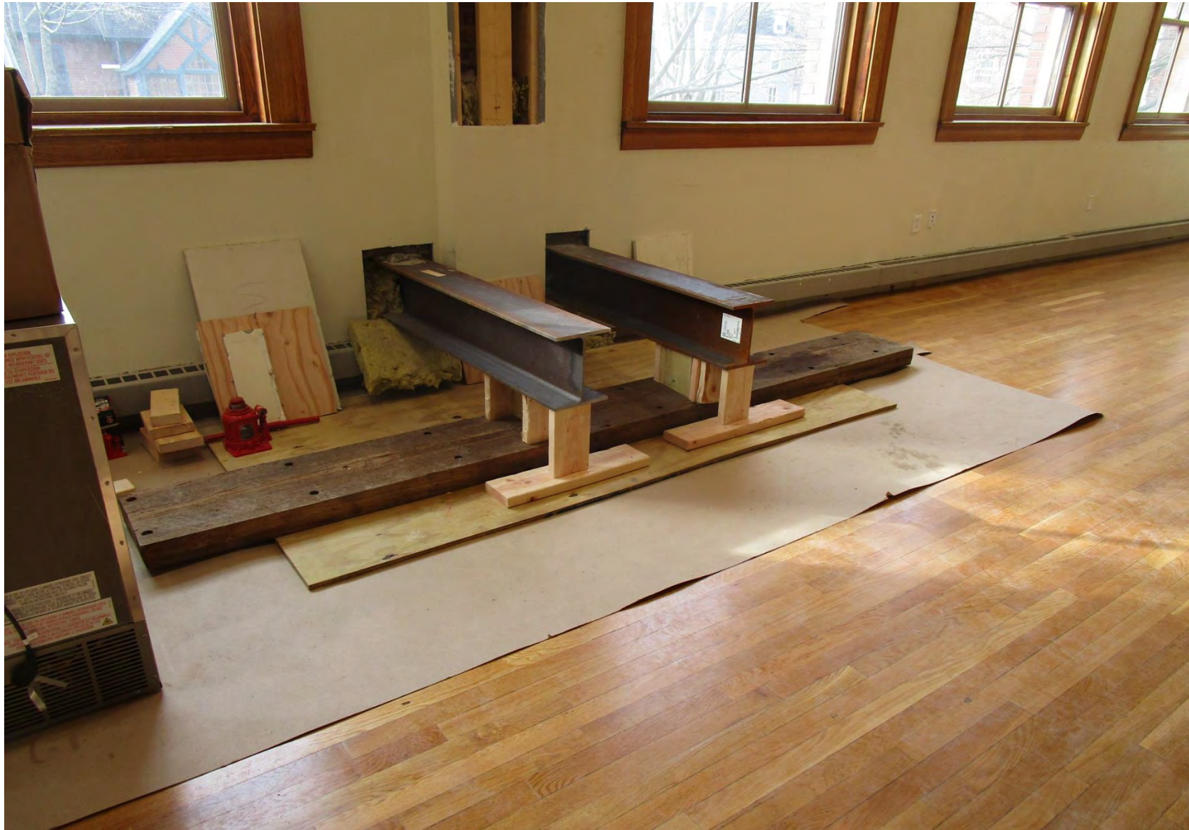
Shoring beams as viewed from the Main Hall.
