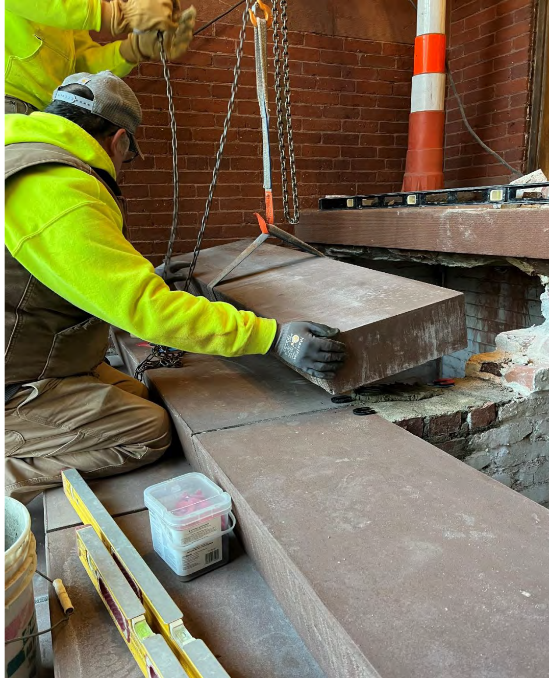
Installation of precast stone stairs
