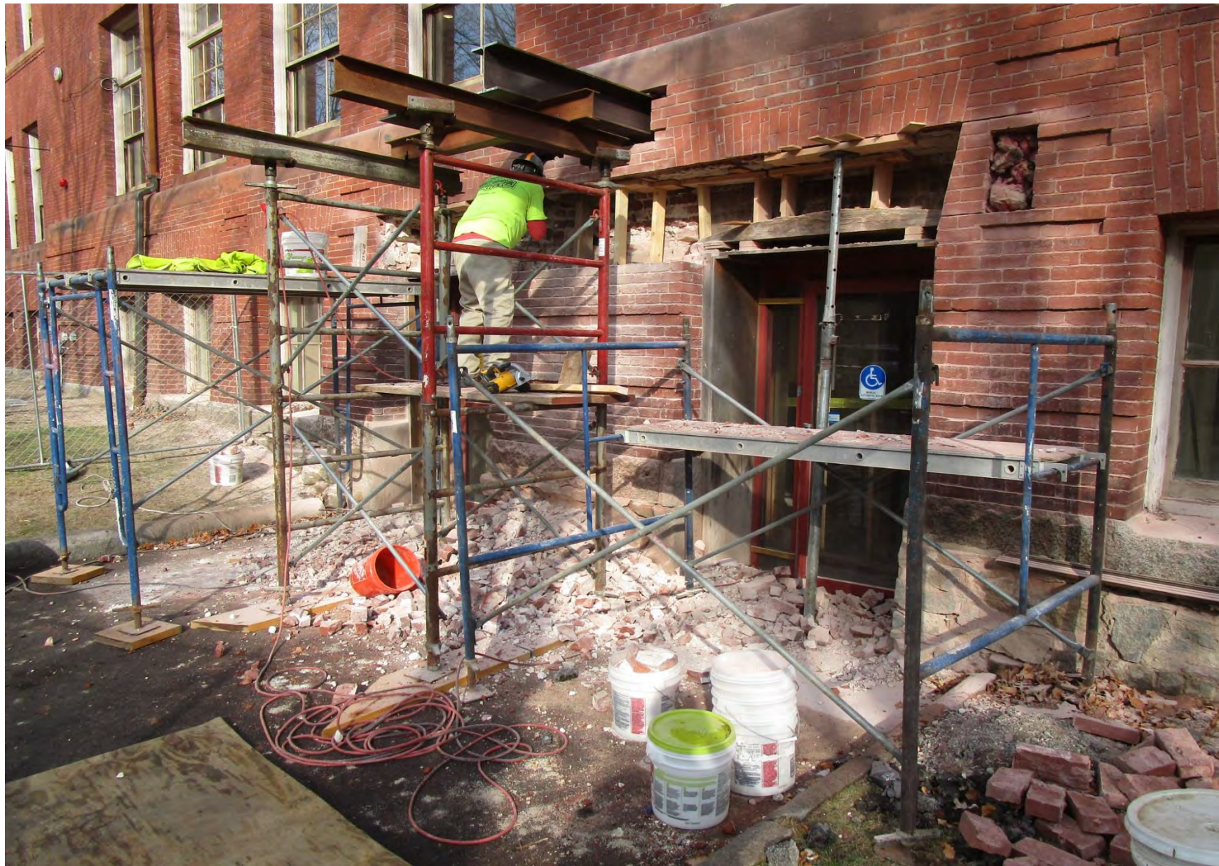
Shoring and demolition of the brick wall at the south entry
