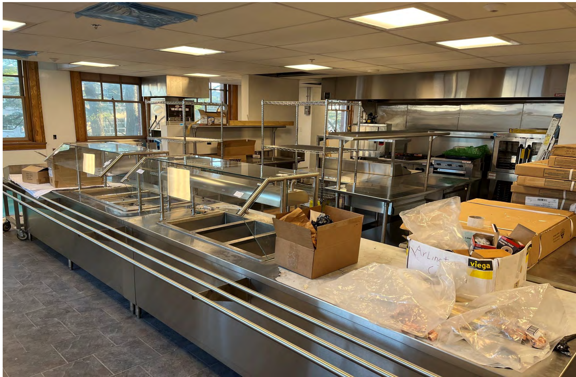
Installation of kitchen serving line and associated food service equipment
