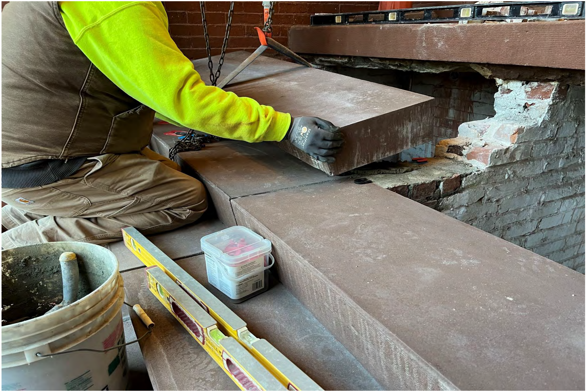
Installation of precast stone stairs
