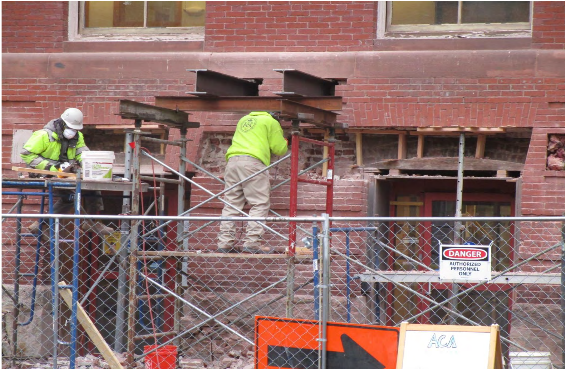
Shoring and demolition of the brick wall at the south entry
