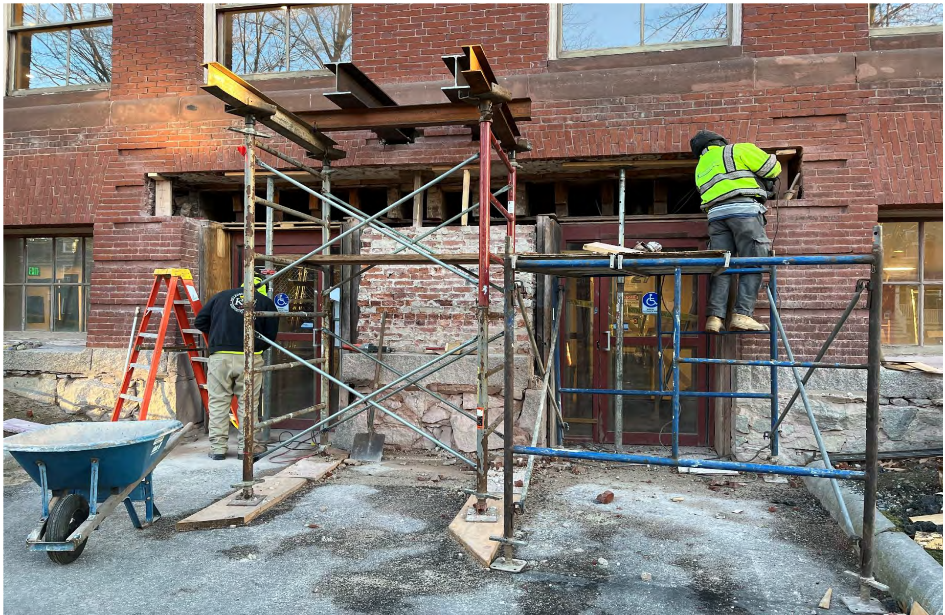
Preparing the wall opening for new structural steel beams
