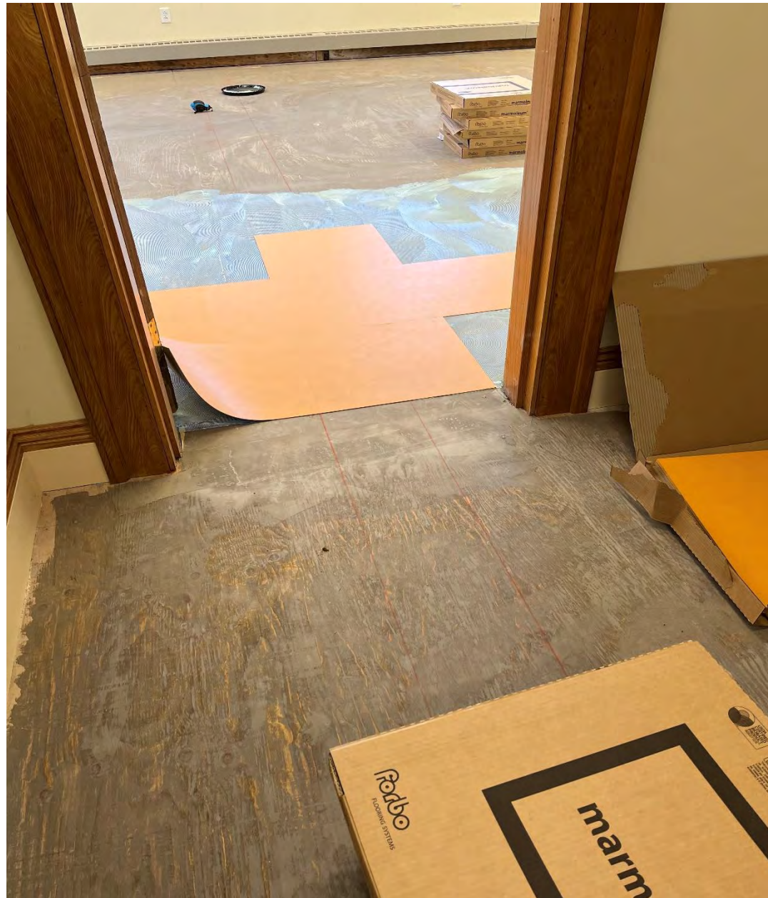
Installation of linoleum tile in Art Room
