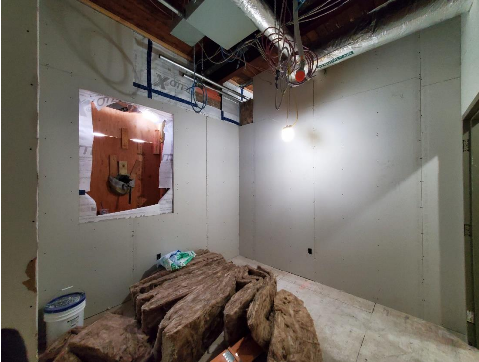
Photo #7 – Building A GWB in Progress (12/15/21)
