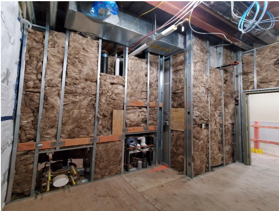
Photo #8 – Building A Framing & Insulation in Progress (12/15/21)
