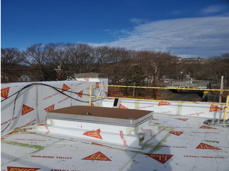
Photo #11 – Building A Roof Hatch Installed (12/14/21)
