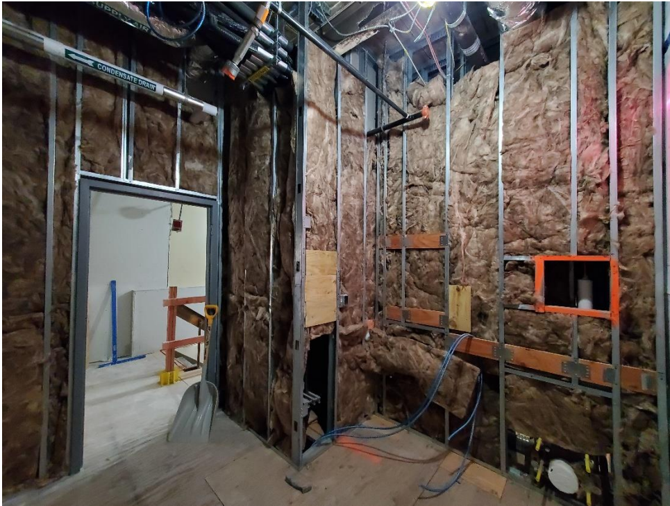
Photo #9 – Building A Framing & Insulation in Progress (12/15/21)
