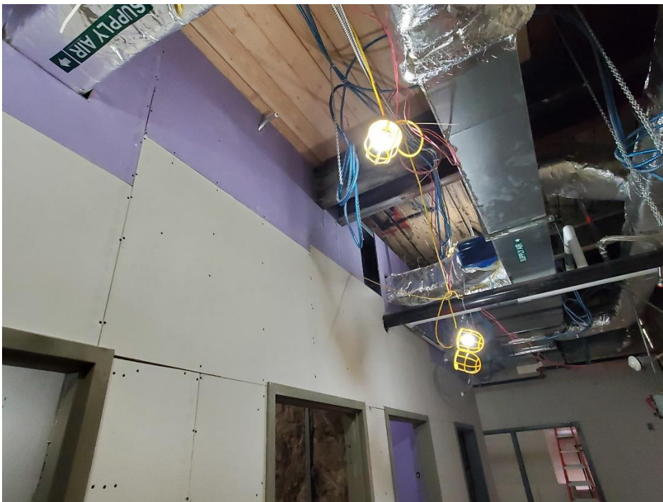
Photo #6 – HVAC Ductwork, Piping and GWB in Progress (12/15/21)
