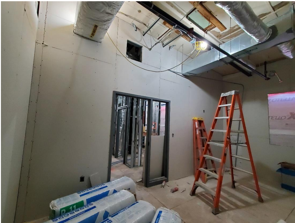
Photo #10 – GWB and MEPFP in Progress (12/14/21)
