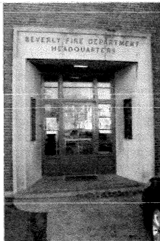
Public entrance on north elevation
