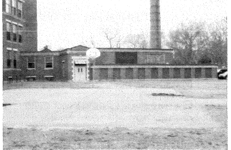
Gymnasium wing on northeast elevation
