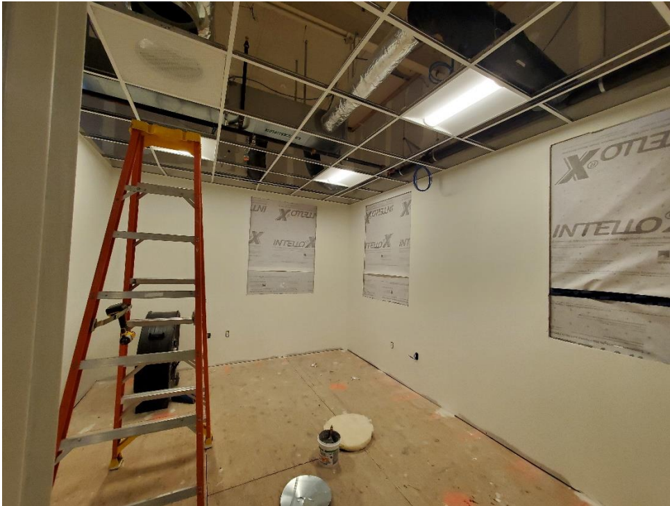
Photo #5 – Building A ACT Ceiling in Progress (1/24/22)
