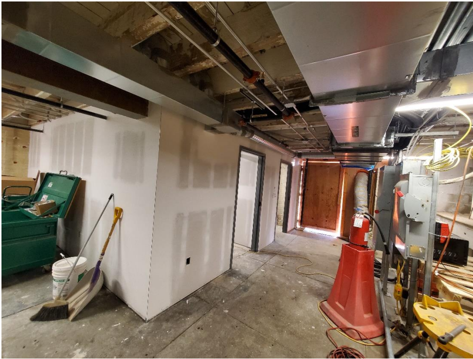
Photo # 1 – Building A in Progress (1/24/2022)
