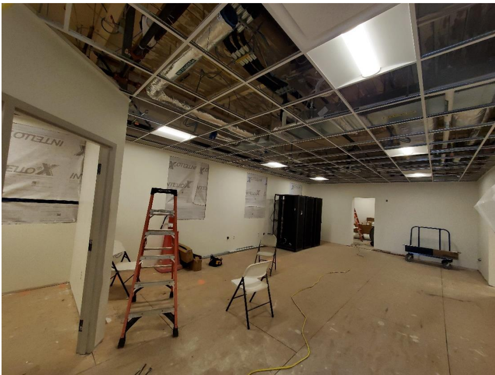
Photo #6 – Building A ACT Ceiling in Progress (1/24/22)
