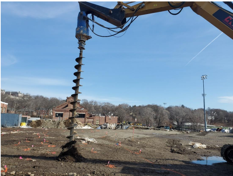
Photo #2 – Ground Improvements in Progress (2/17/22)
