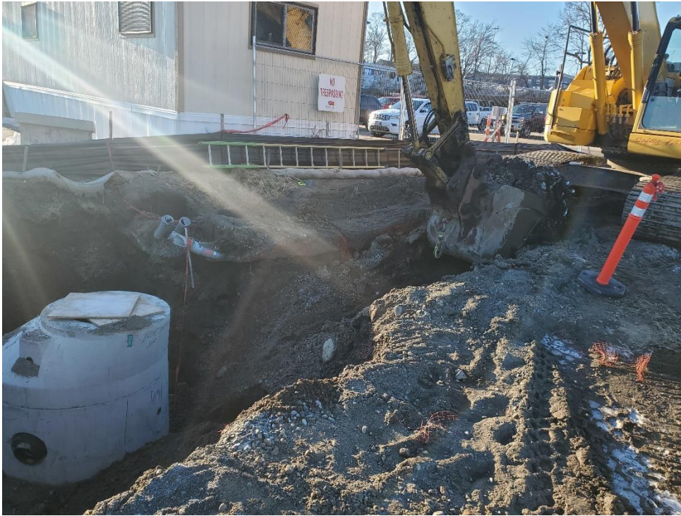
Photo # 1 – Drainage Structure in Progress (2/11/2022)
