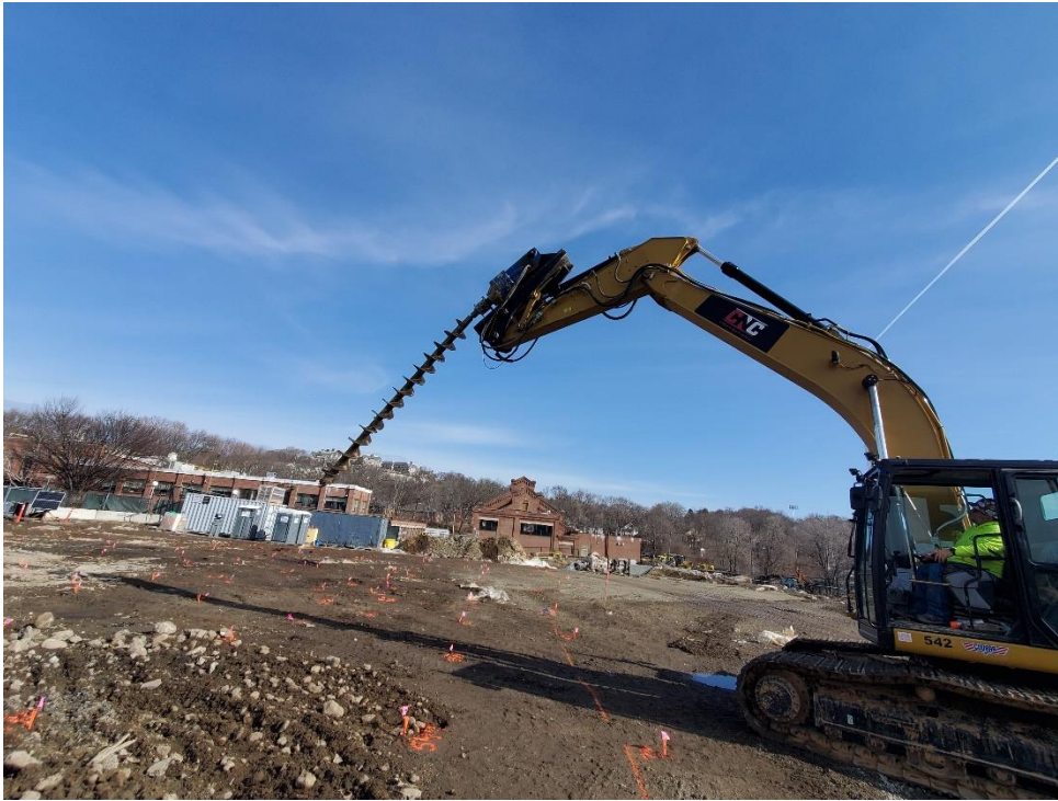
Photo #3 – Ground Improvements in Progress (2/17/22)
