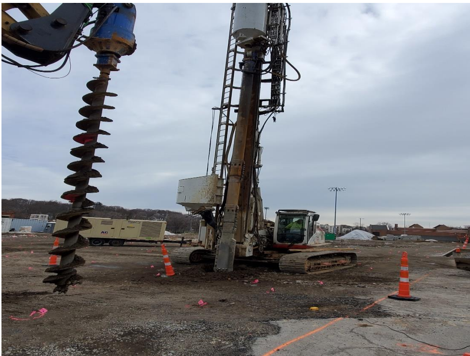
Photo #6 – Ground Improvements in Progress (2/24/22)
