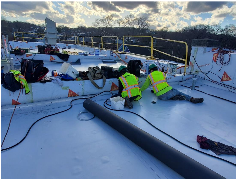
Photo # 4 – Roofing at Building A (2/23/2022)
