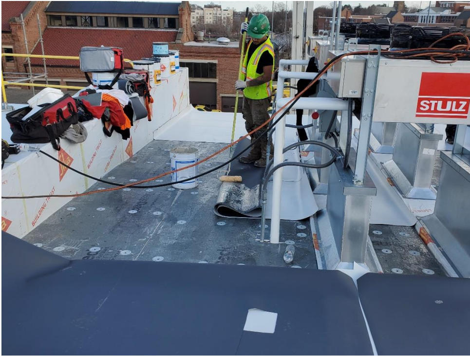
Photo #5 – Roofing at Building A (2/23/22)
