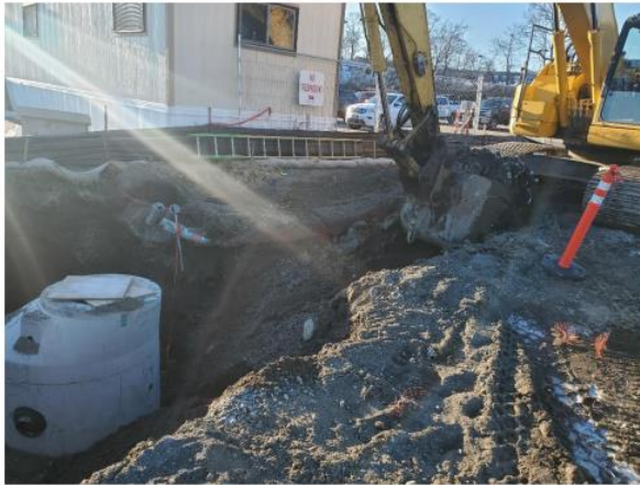
Photo # 1 – Drainage Structure in Progress (2/11/2022)
