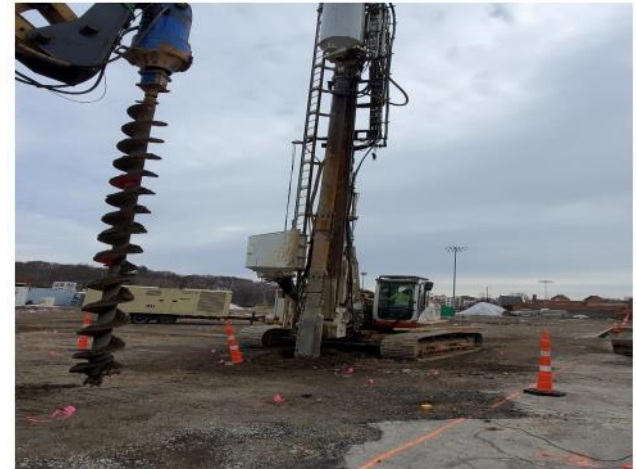
Photo #6 – Ground Improvements in Progress (2/24/22)
