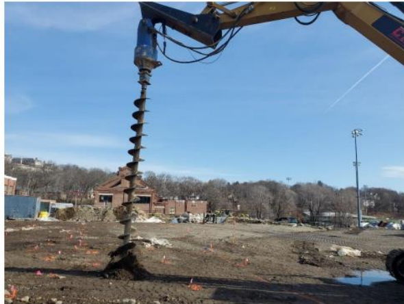
Photo #2 – Ground Improvements in Progress (2/17/22)
