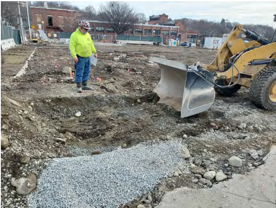
Photo #4 – Sitework in Progress (3/7/22)
