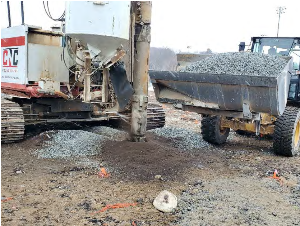
Photo #6 – Ground Improvements in Progress (3/9/22)
