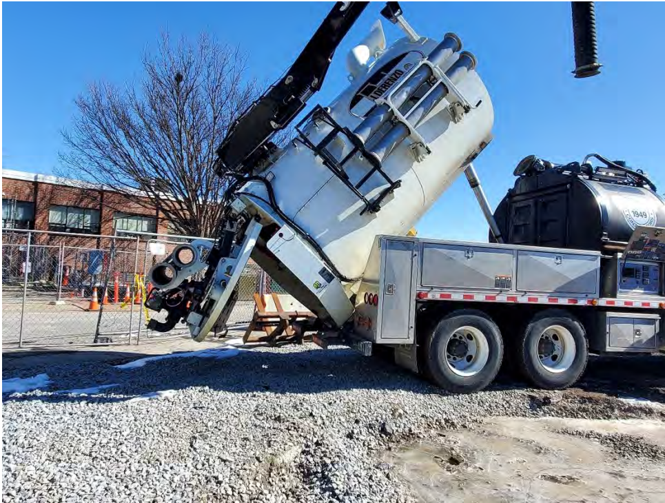
Photo #3 – Sitework in Progress (3/4/22)
