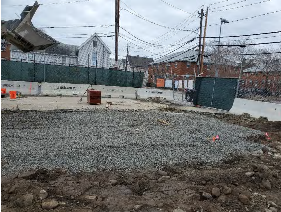
Photo #5 – Sitework in Progress (3/7/22)
