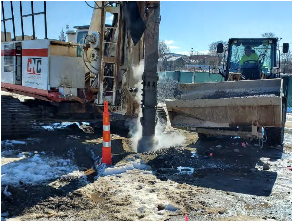
Photo #1 – Ground Improvements in Progress (3/2/2022)
