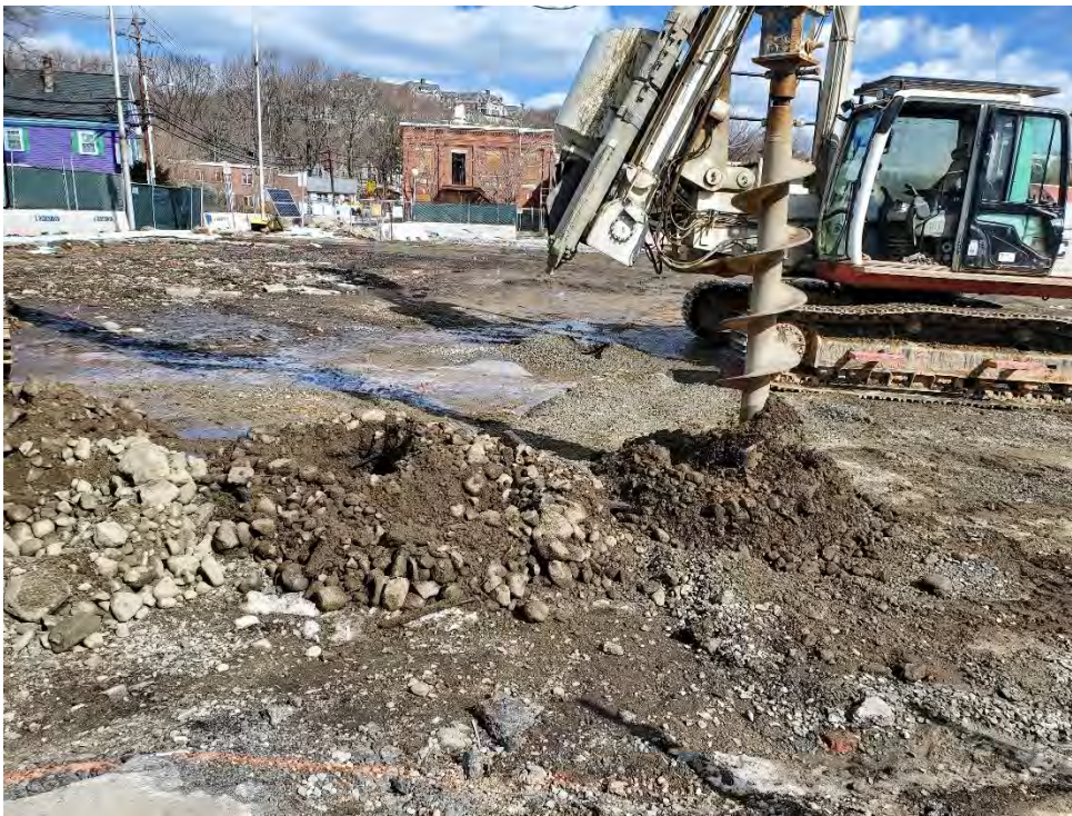
Photo #2 – Ground Improvements in Progress (3/3/22)
