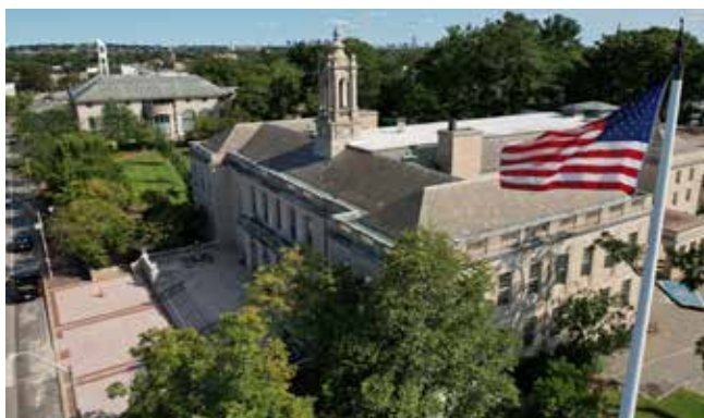
Restored Town Hall Plaza.
