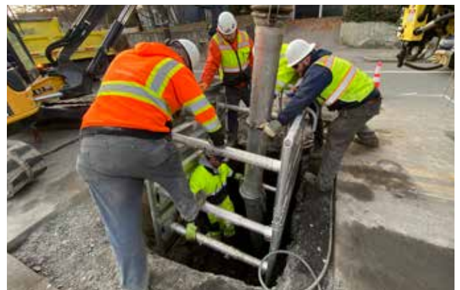
Water Division performing water main work.
