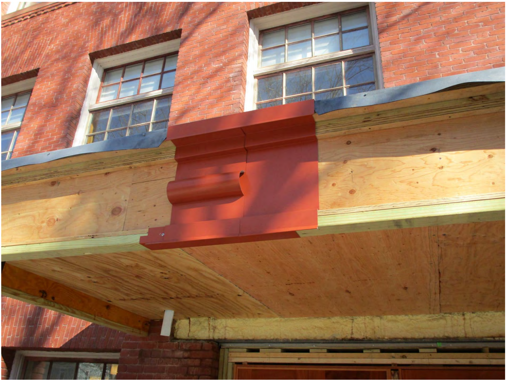
Maple Street entrance canopy sheetmetal edge mockup
