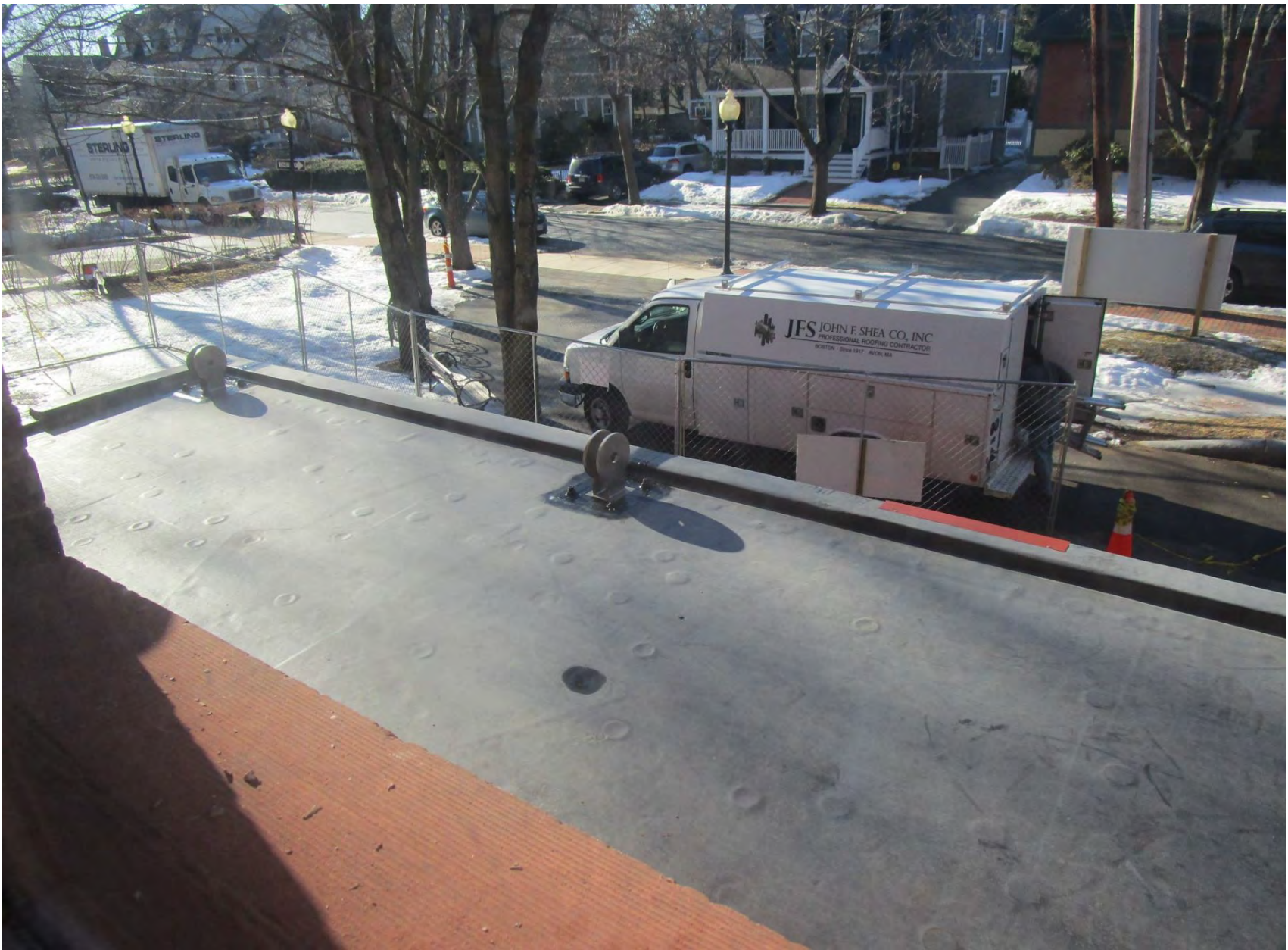
Maple Street entrance canopy EPDM roof
