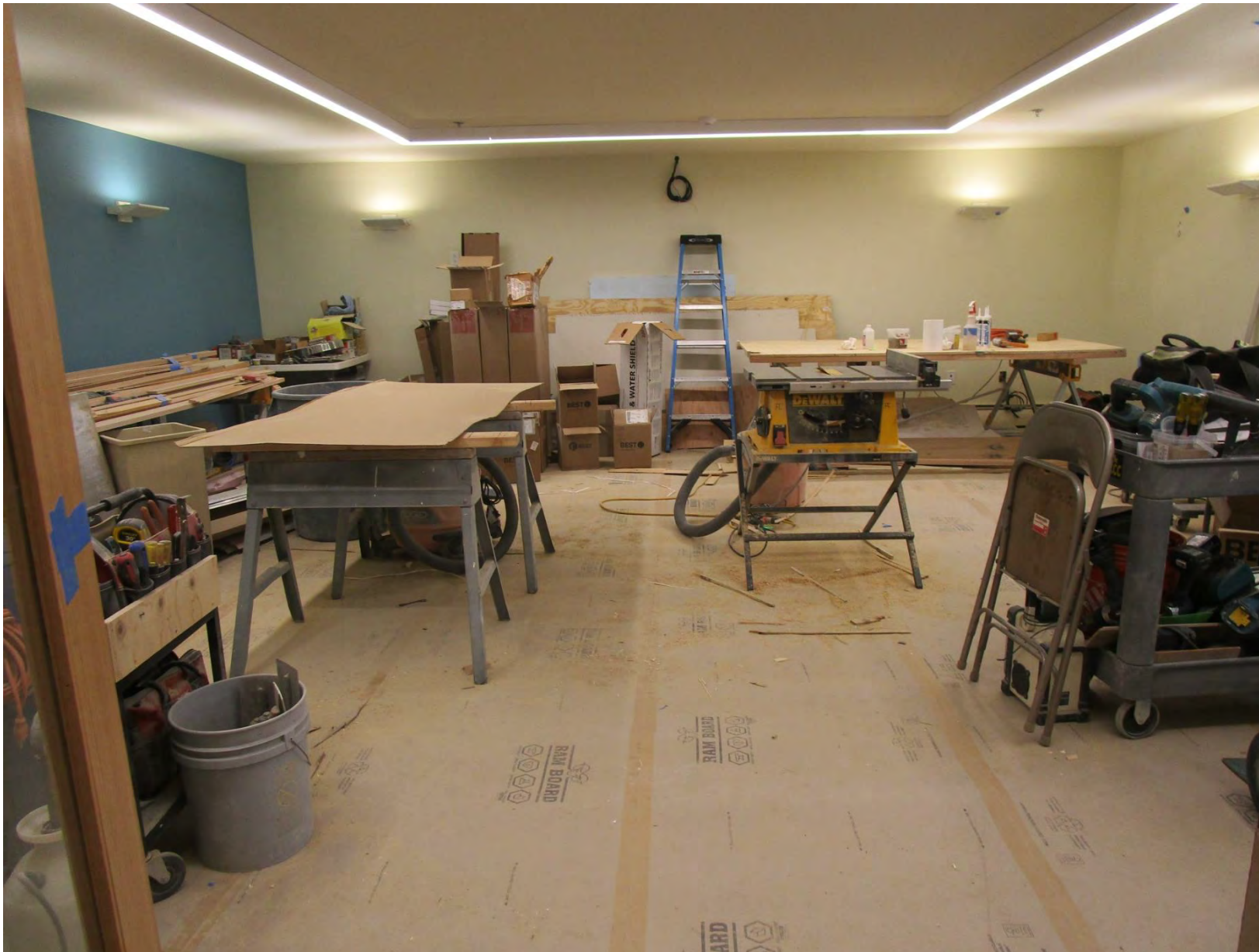
Exercise room retained by KSR as a shop area
