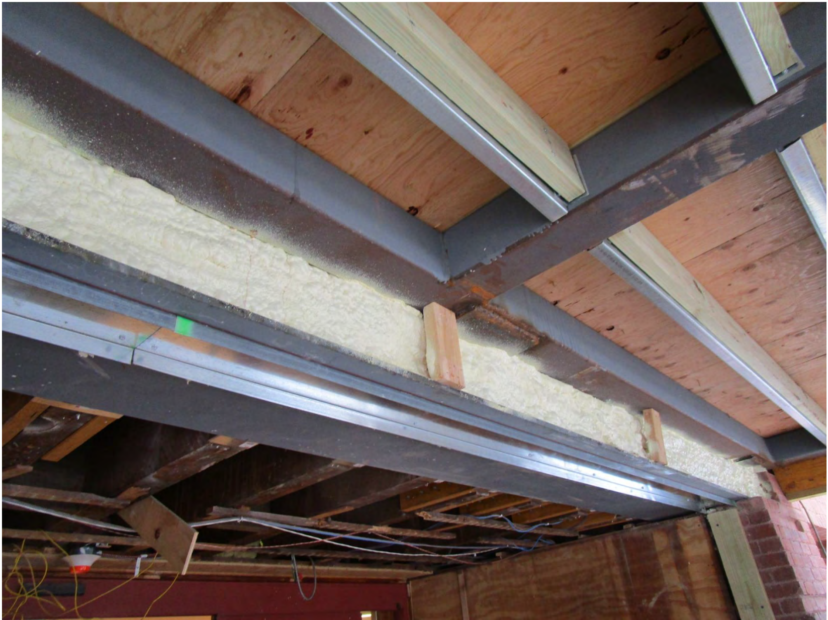
Maple Street entrance canopy framing with spray foam insulation at beams
