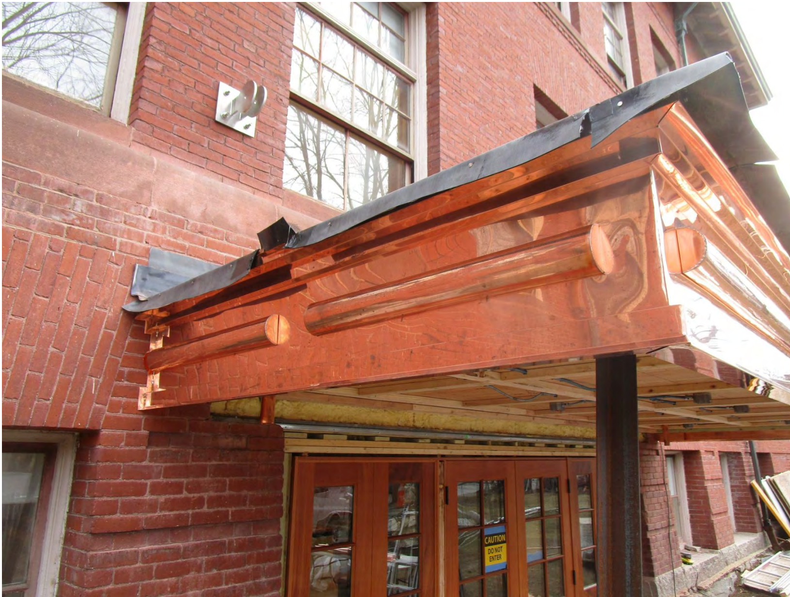
Maple Street entry canopy with copper edge metal
