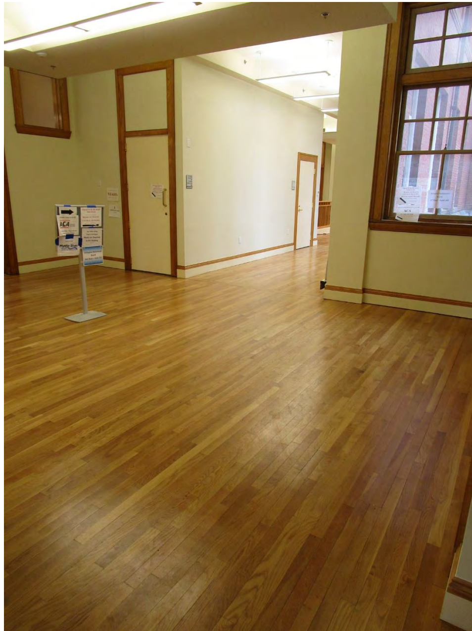
East entry lobby with finished hardwood floor
