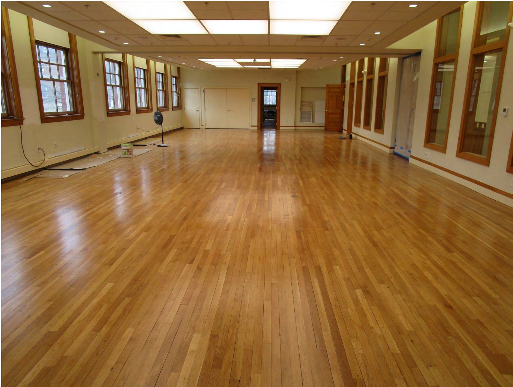
Finished hardwood floor in Main Hall Rooms 118/119
