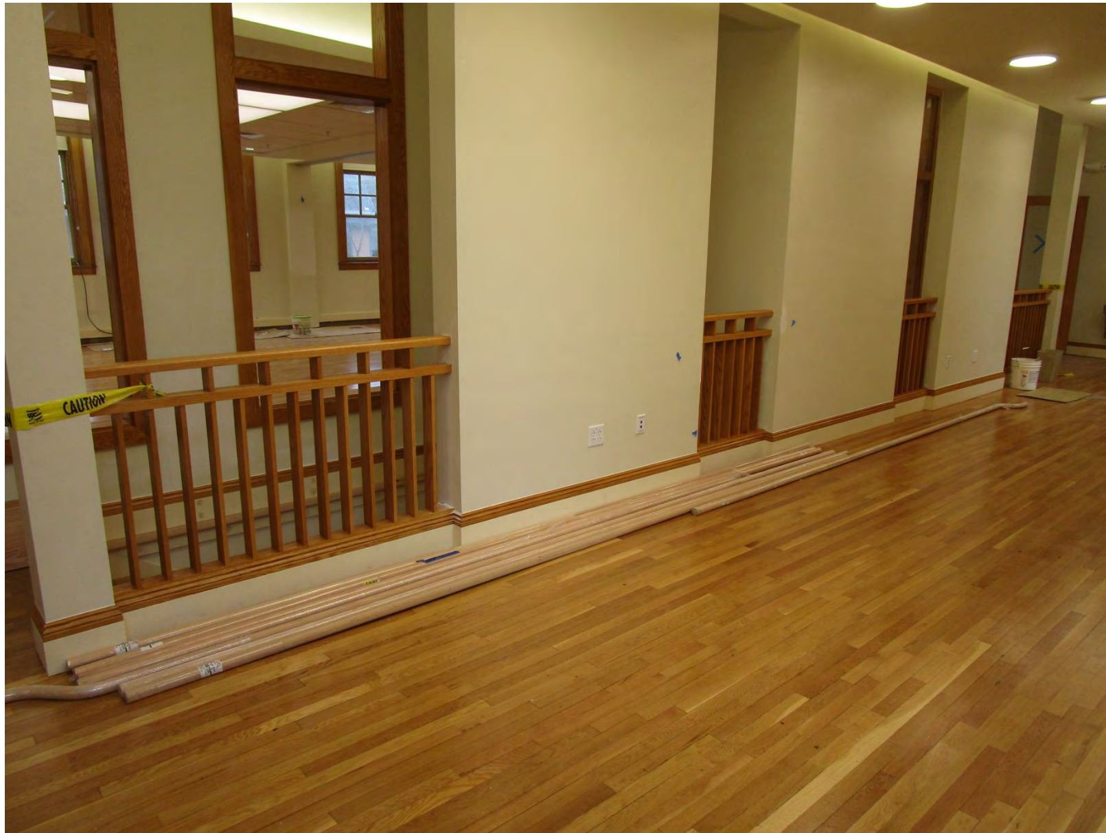
Stair #3 rails at gallery
