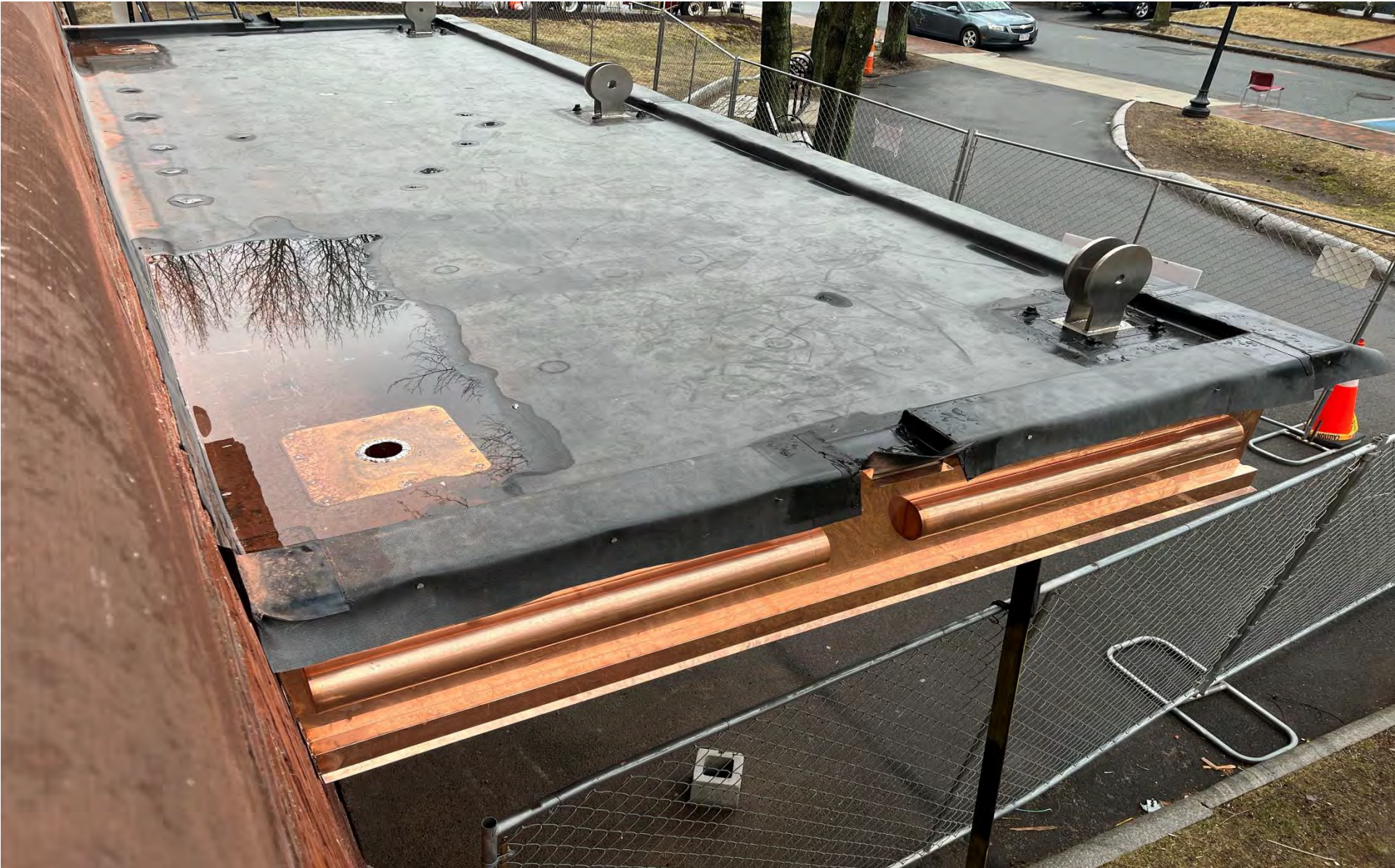
Maple Street entry canopy roof with copper
