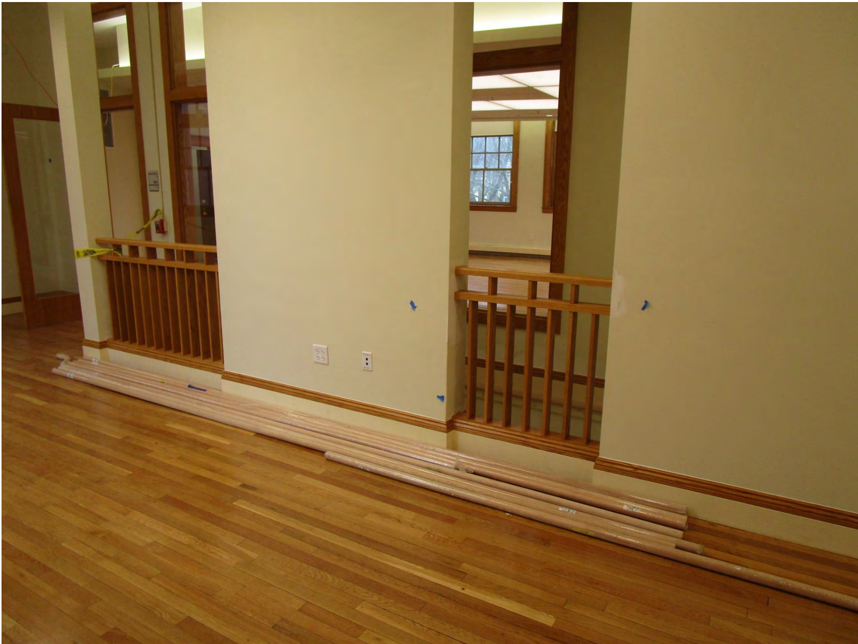
Stair #3 rails at gallery
