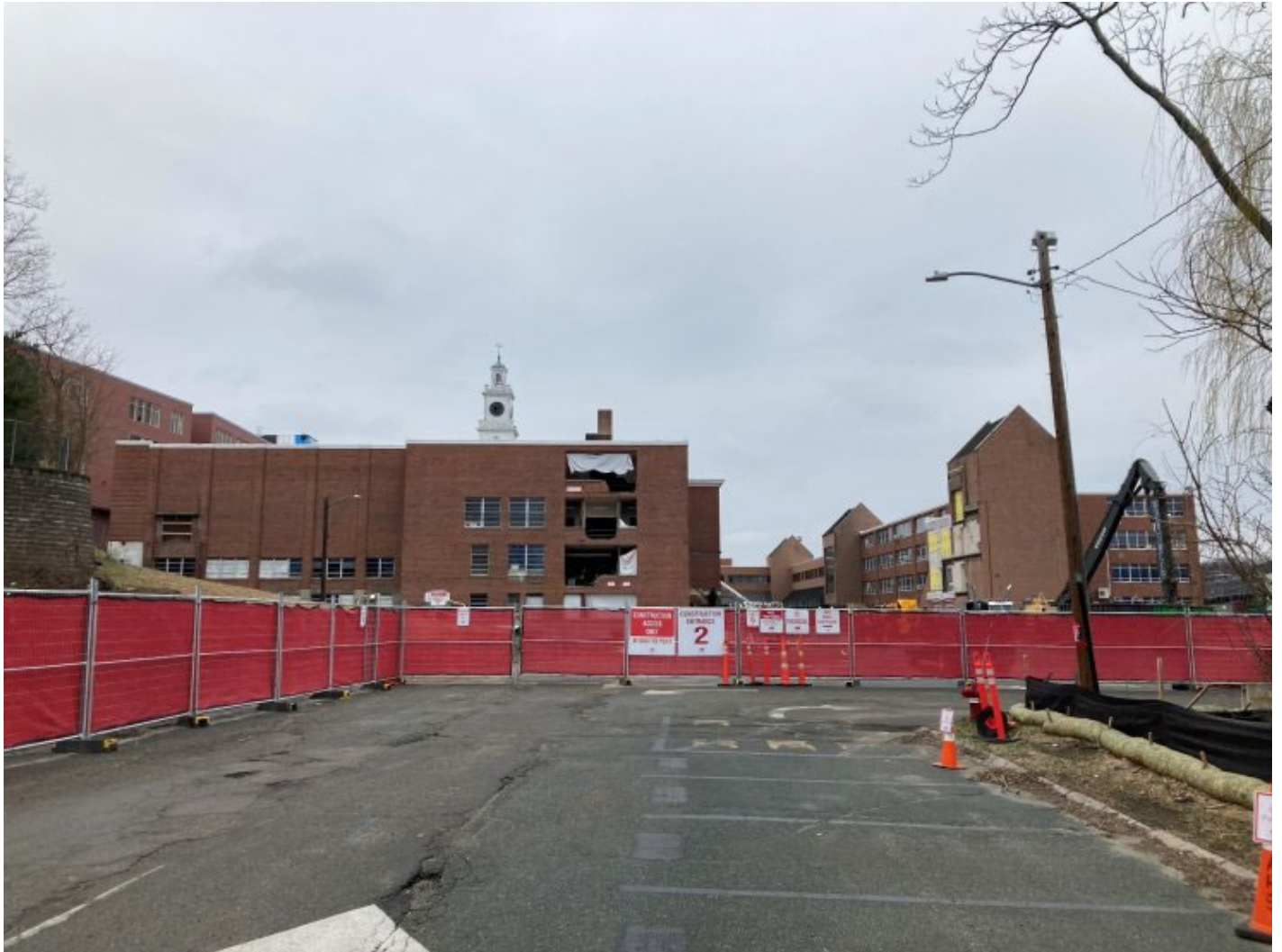
Photograph 5: Collomb Building East Elevation
