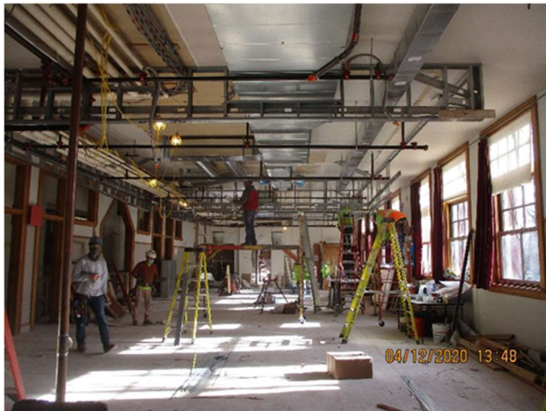
Installation of new beam and heating and cooling ducts, and new movable partition
