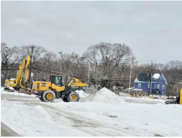
Removing snow to enable site work to continue
