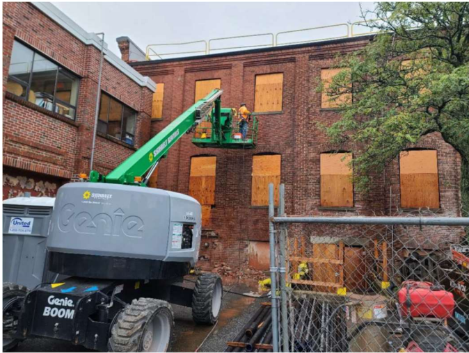
Cleaning of brick and mortar
