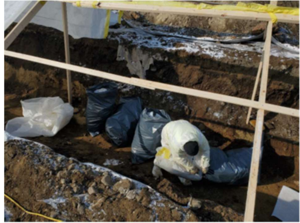
Abatement of asbestos-covered pipes
