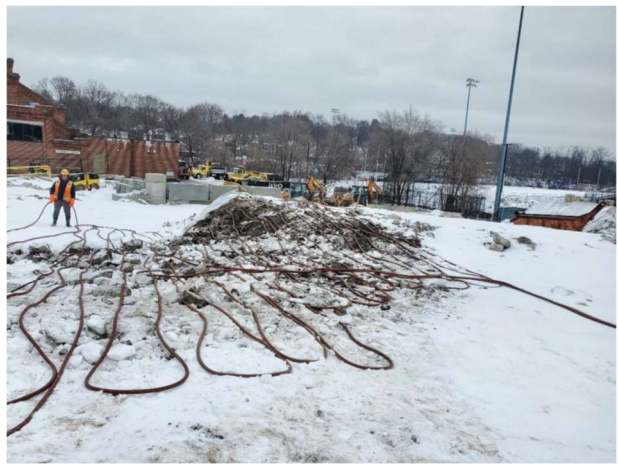
Thawing the soil for site work
