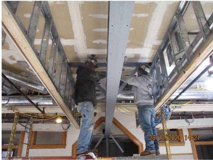
Installation of new beam and heating and cooling ducts, and new movable partition
