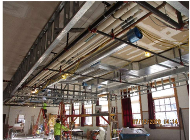
Installation of new beam and heating and cooling ducts, and new movable partition
