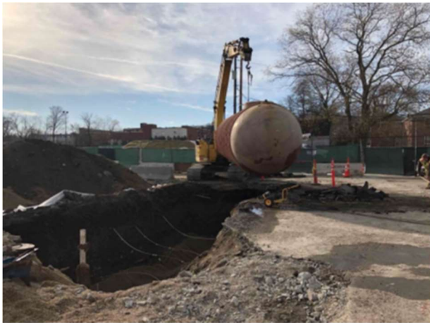
Removal of gas storage tank
