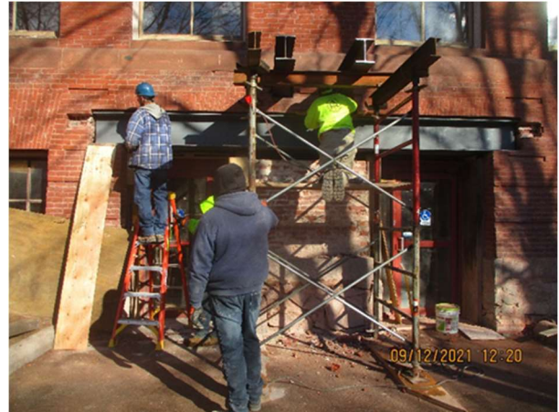
Removal of brick, installation of new beam and canopy
