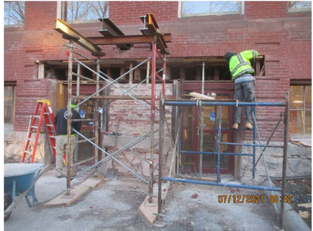
Removal of brick, installation of new beam and canopy
