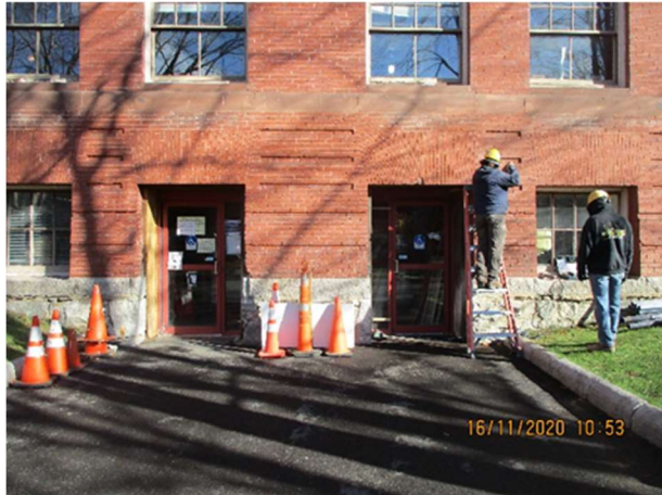
Removal of brick, installation of new beam and canopy
