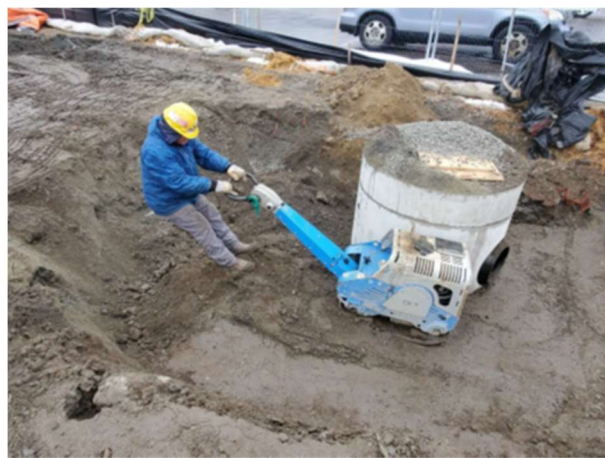
Installation of site drainage structures
