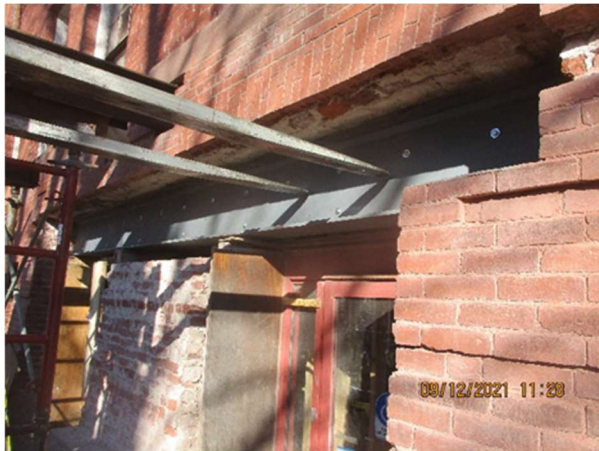
Removal of brick, installation of new beam and canopy
