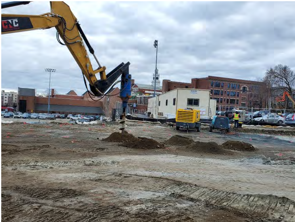
Photo #4 – Ground Improvements in Progress (4/7/22)
