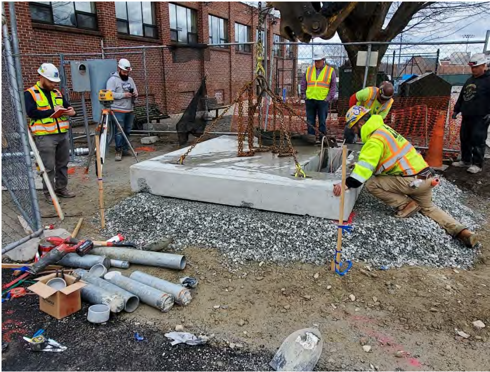
Photo #5 – Electrical Transformer Pad in Progress (4/8/22)
