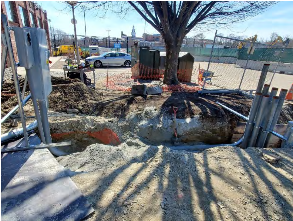
Photo # 3 – Utility Work in Progress (4/5/2022)
