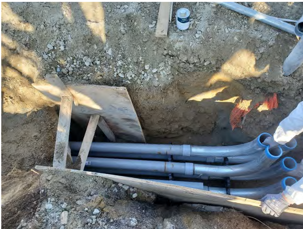
Photo # 2 – Utility Work in Progress (4/5/2022)
