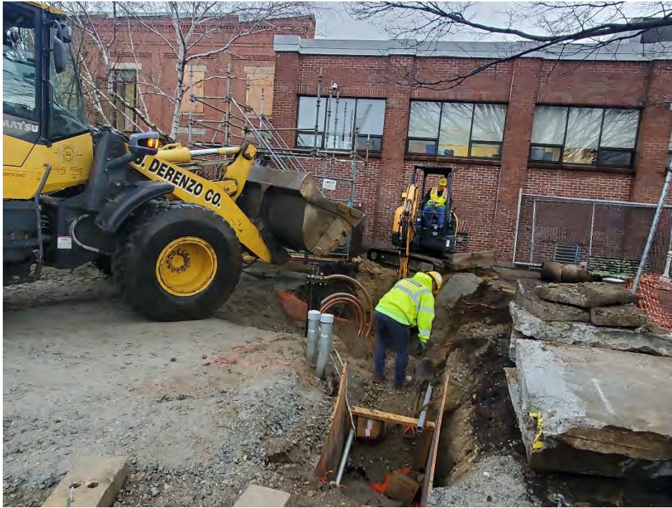
Photo # 1 – Electrical Ductbank in Progress (4/1/2022)
