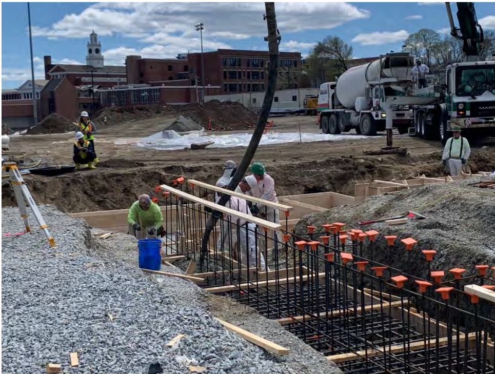
Photo #6 – First Concrete Footing Pour in Progress (4/20/22)
