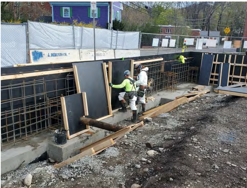
Photo #8 – Forming of Foundation Walls in Progress
