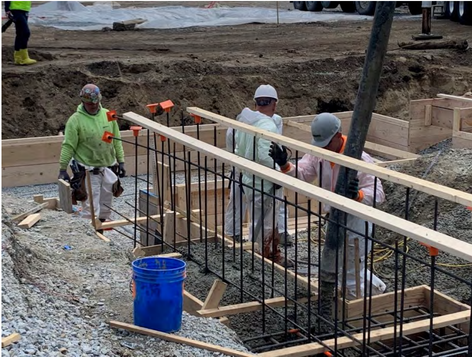
Photo #7 – First Concrete Footing Pour in Progress
