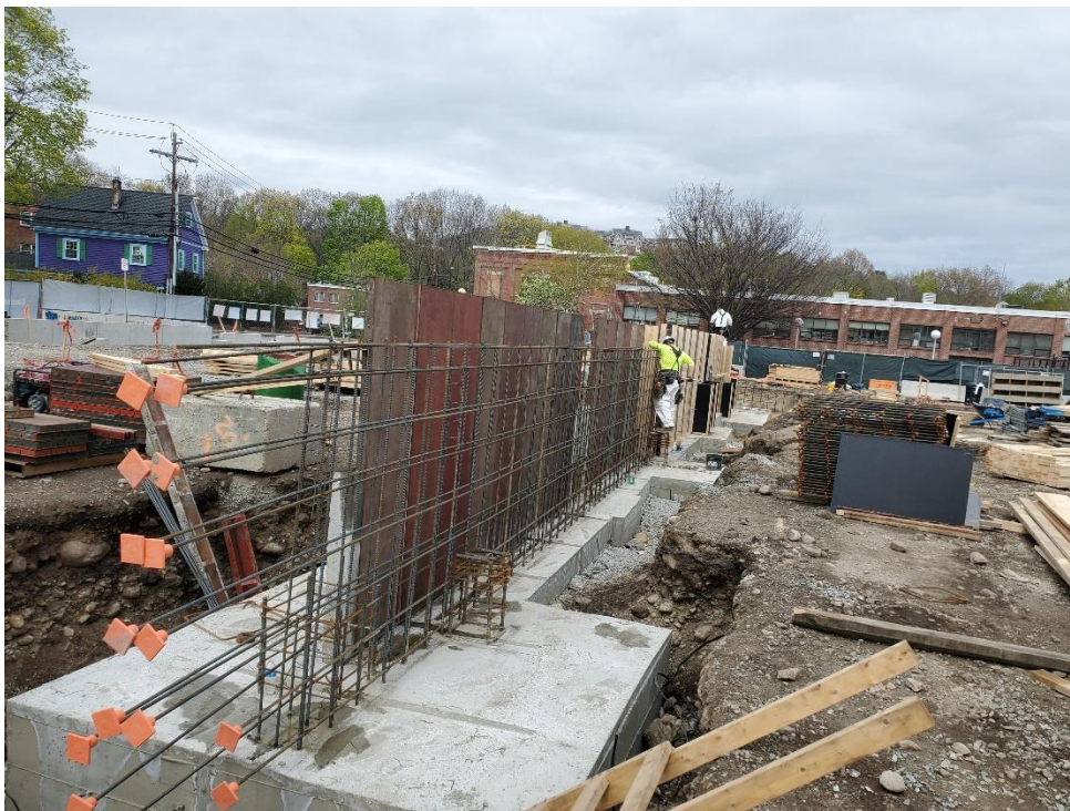
Photo # 2 – Rebar and Foundation Wall in Progress (5/3/2022)
