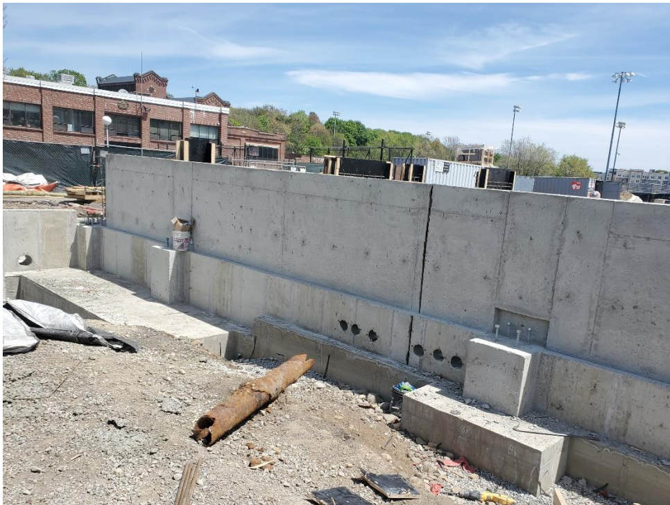
Photo #4 – Foundation Wall Complete (5/9/22)
