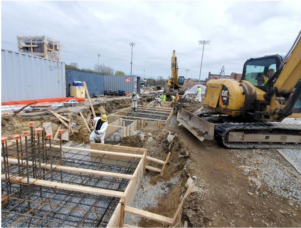
Photo # 1 – Footings in Progress (5/3/2022)
