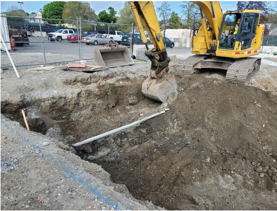
Photo #8 – Excavation in Progress (5/11/22)
