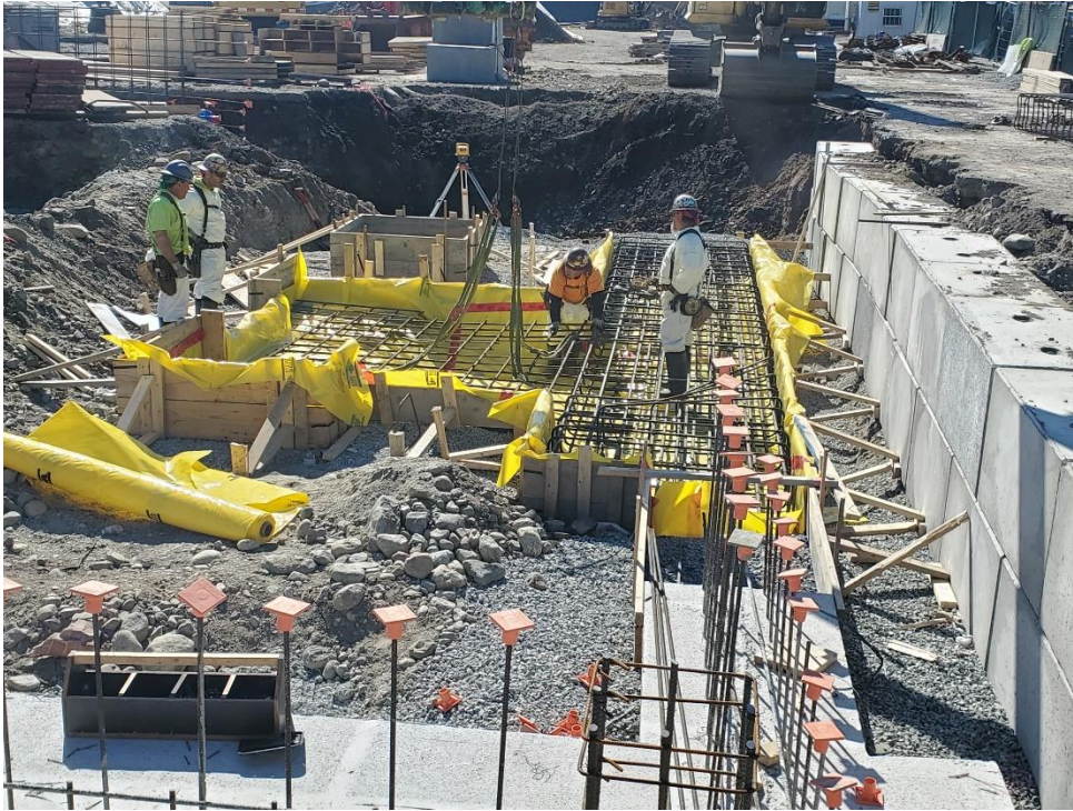
Photo #5 – Rebar and Foundation Wall in Progress (5/10/22)
