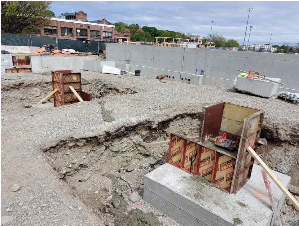
Photo #6 – Interior Footings in Progress (5/11/22)
