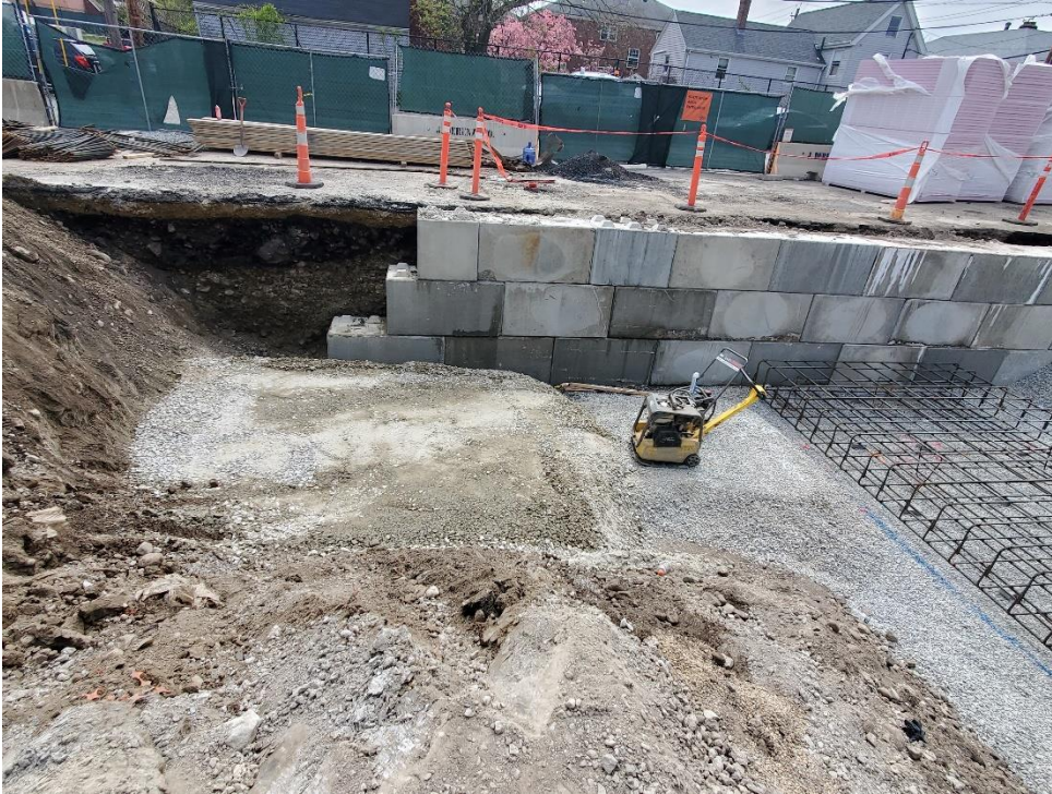
Photo #7 – Compaction in Progress (5/11/22)
