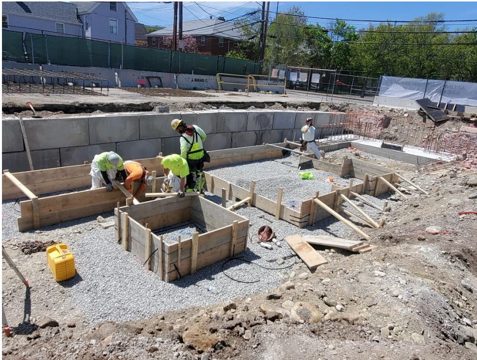
Photo # 3 – Interior Footings in Progress (5/9/2022)
