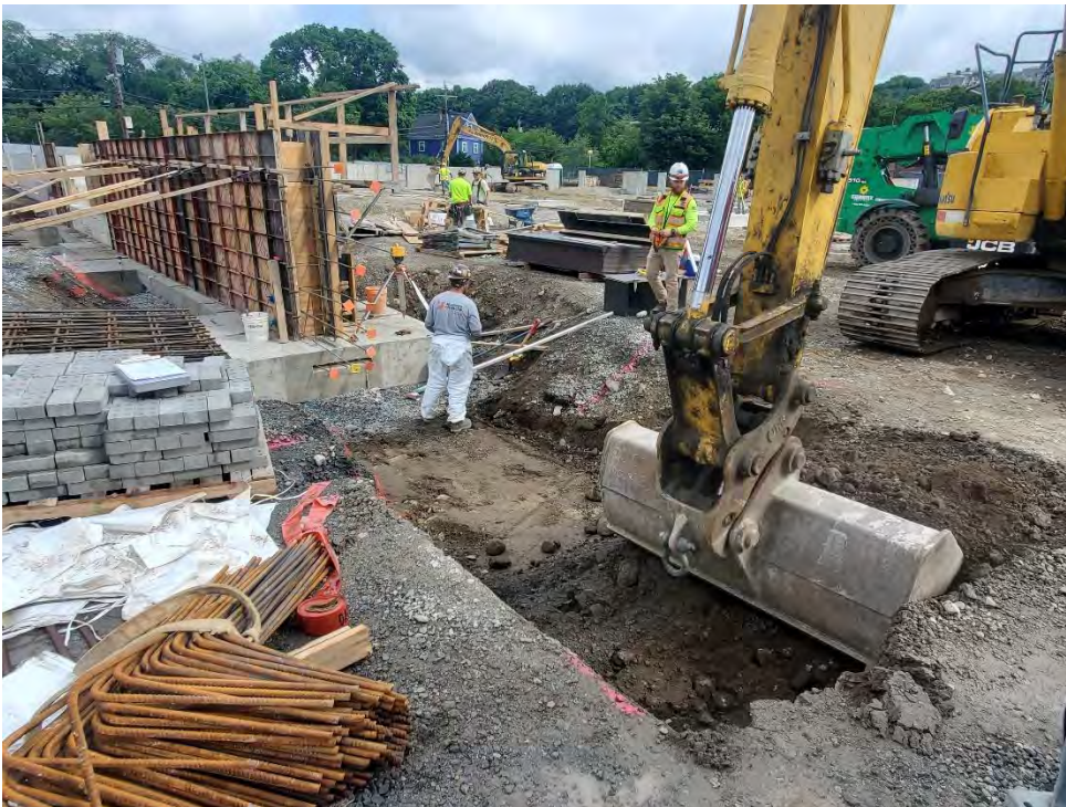
Photo # 4 – Foundations and Footings in Progress (6/13/2022)
