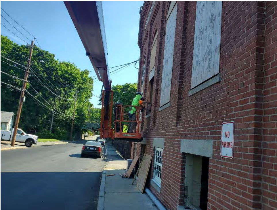
Photo # 2 – Building A Window Installation in Progress (6/7/2022)
