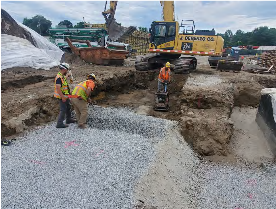
Photo #5 – Sitework in Progress (6/16/22)
