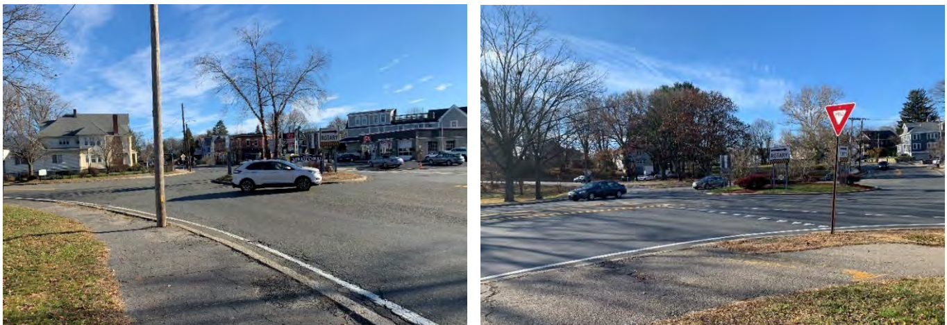
Figure 17 (Left) Excess pavement and lack of horizontal deflection at the High Street rotary; (right) no crossing on the path side of the Medford Street rotary
