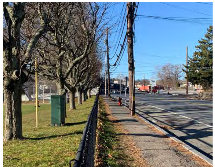
Figure 27: Looking west on Summer Street along the narrow sidewalk with utility poles adjacent to a chain link fence and Buzzell Field. Recommendations in this chapter detail the path as it responds to the changing character of the corridor.
