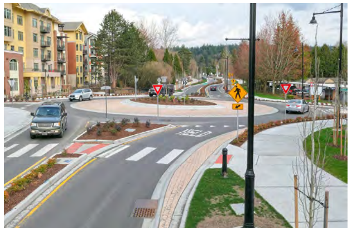
Figure 13: Example of a Modern Roundabout
