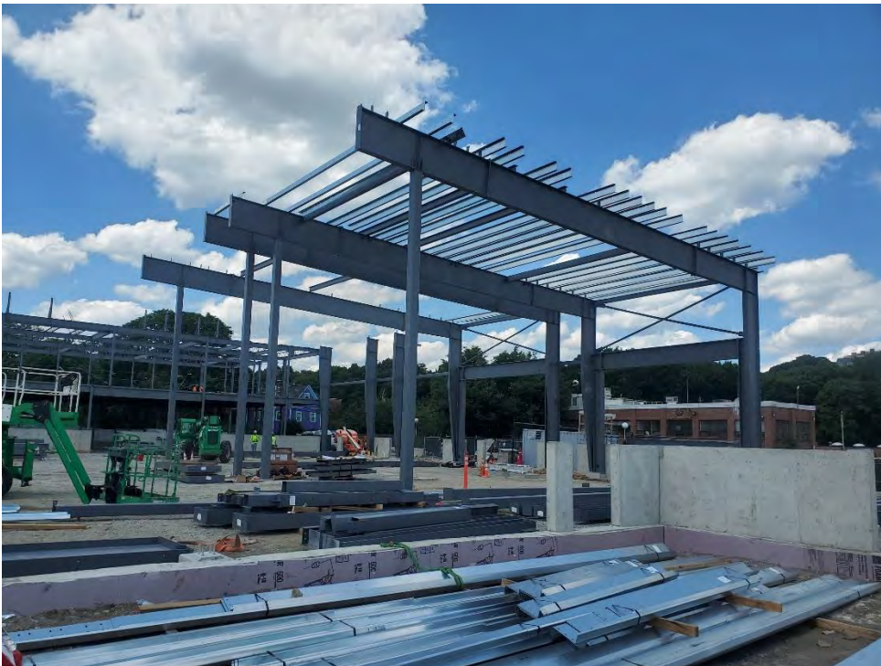
Photo #6 – Building E Steel Erection in Progress (7/13/22)
