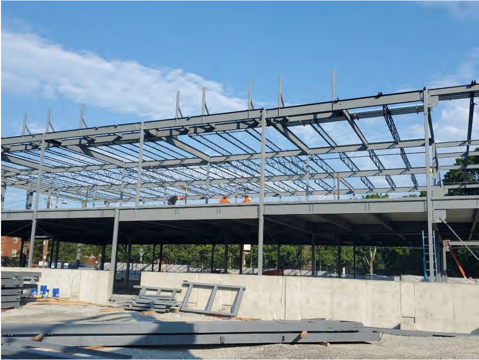
Photo # 1 – Building E Steel Erection in Progress (7/12/22)
