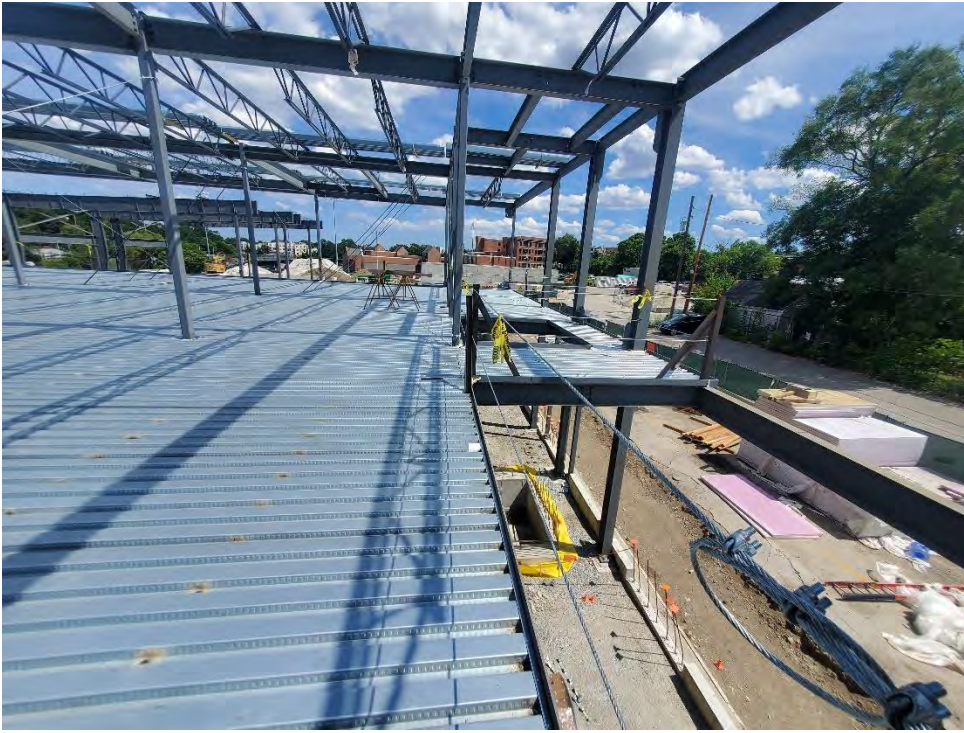
Photo #5 – Building E Steel Erection in Progress (7/13/22)
