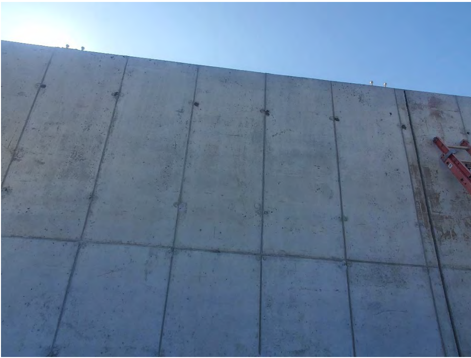
Photo # 4 – Salt Shed Foundation Walls in Progress (7/13/22)
