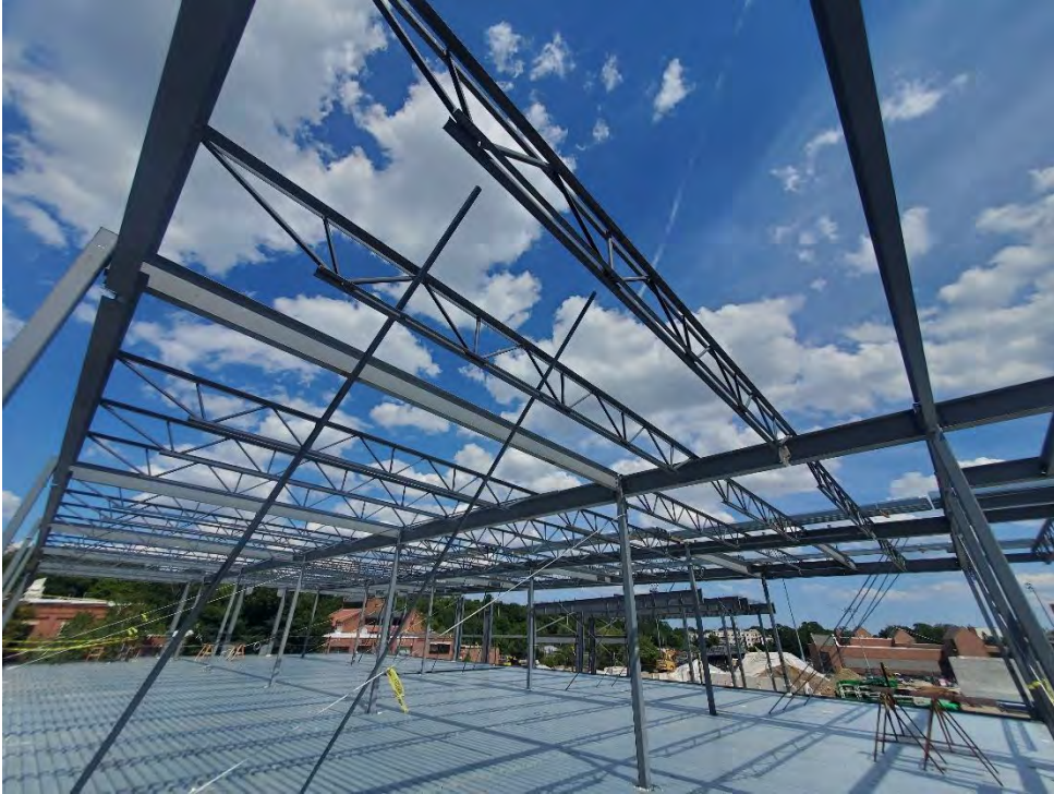
Photo # 3 – Building E Steel Erection in Progress (7/13/22)
