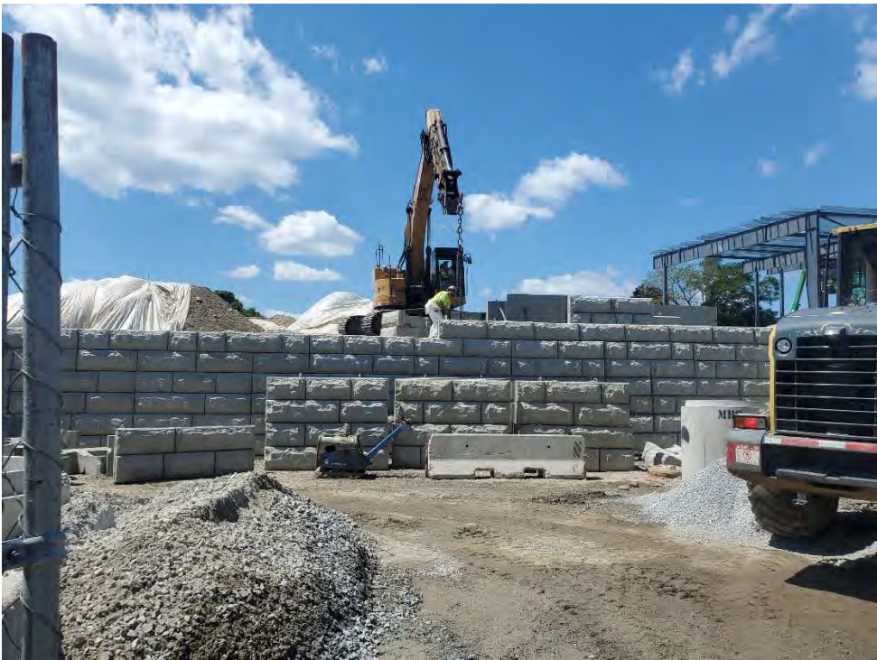
Photo # 2 – Retaining Wall in Progress (7/13/22)
