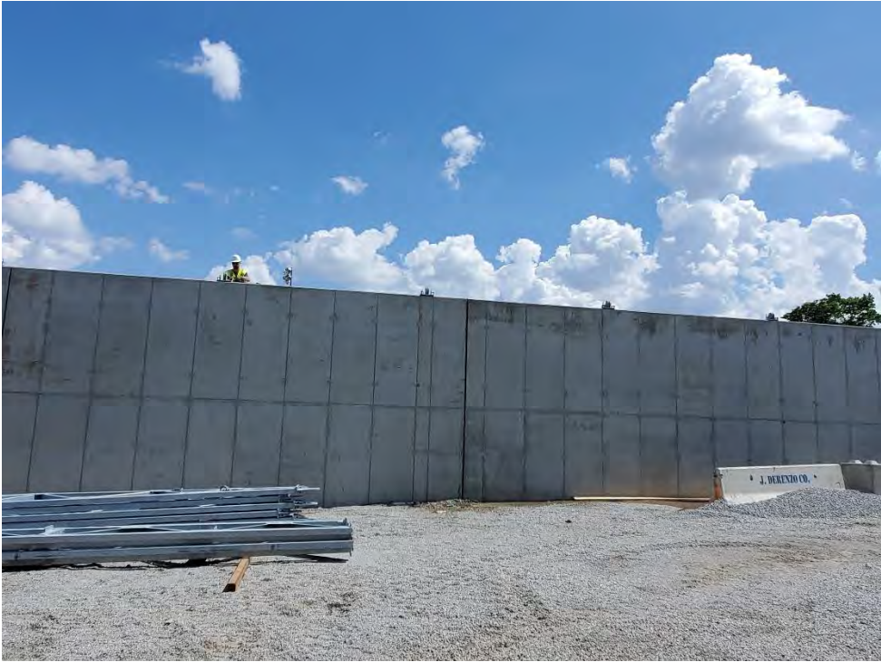
Photo # 1 – Salt Shed in Progress (8/8/22)
