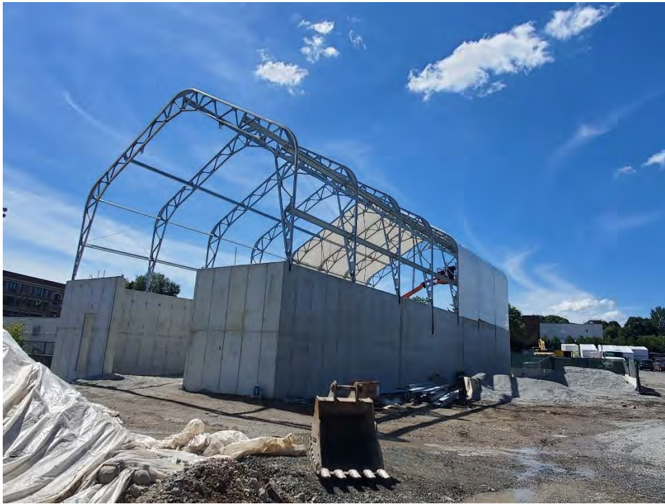
Photo #5 – Salt Shed Roof Canopy in Progress (8/16/22)
