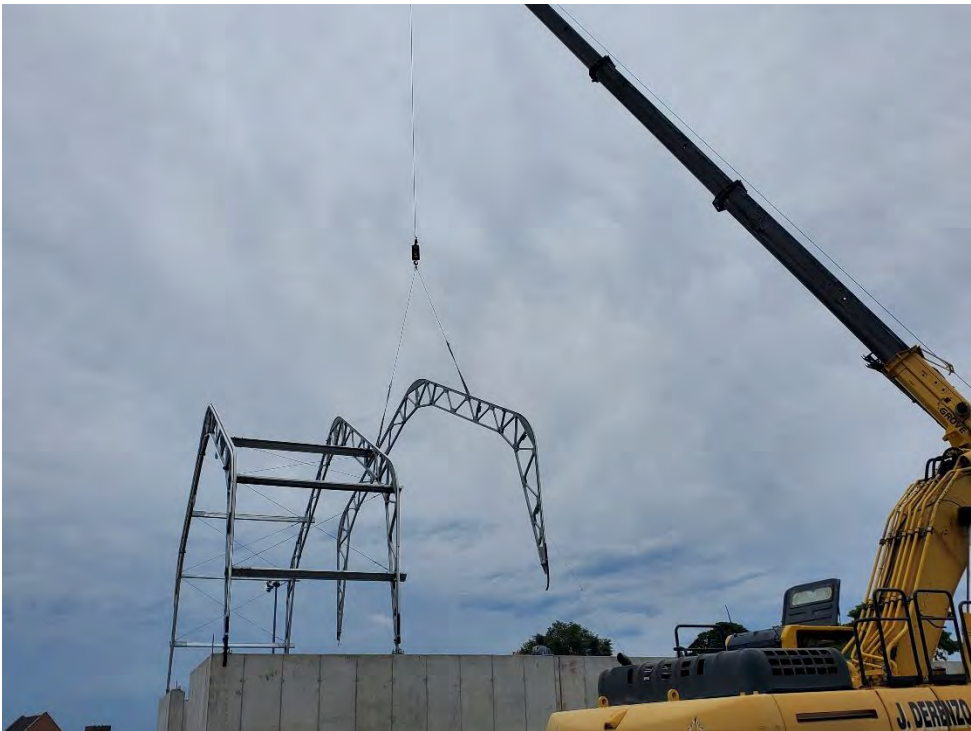
Photo # 2 – Salt Shed Canopy Roof Frame in Progress (8/11/22)
