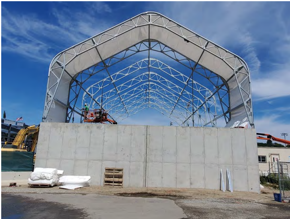
Photo #6 – Salt Shed Roof Canopy in Progress (8/16/22)
