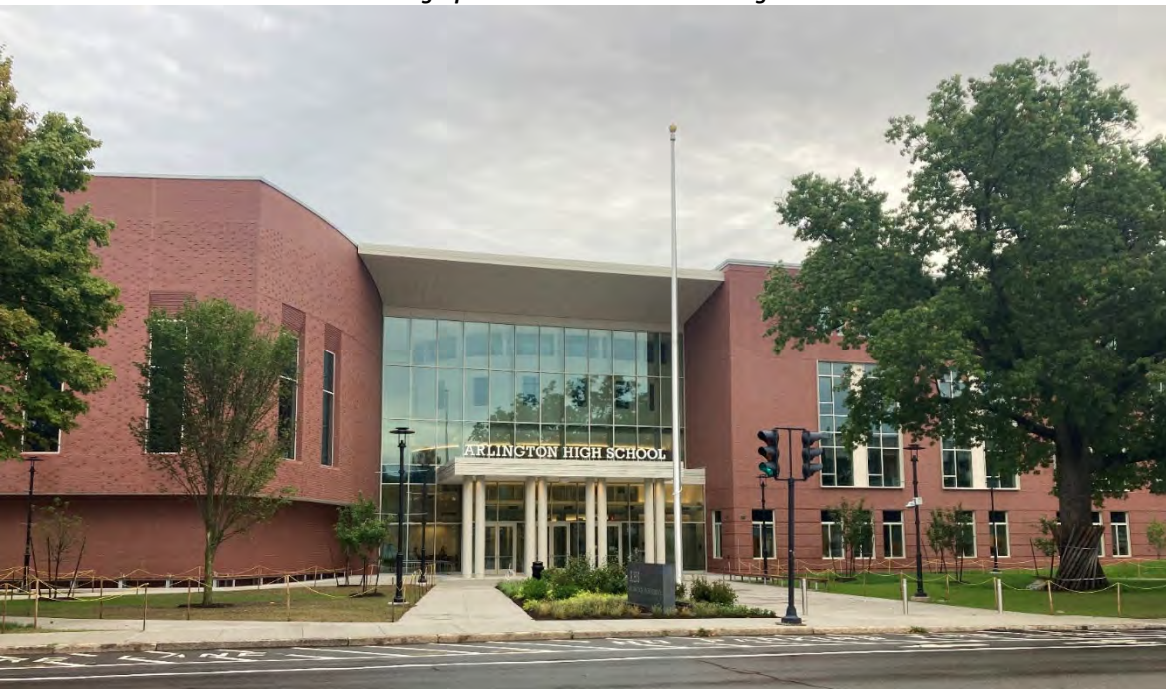
Photograph 2: Building D/E South Elevation (Main Entrance #1)
