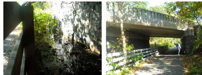
Figure 67. Existing images of Lowell Street Underpass
