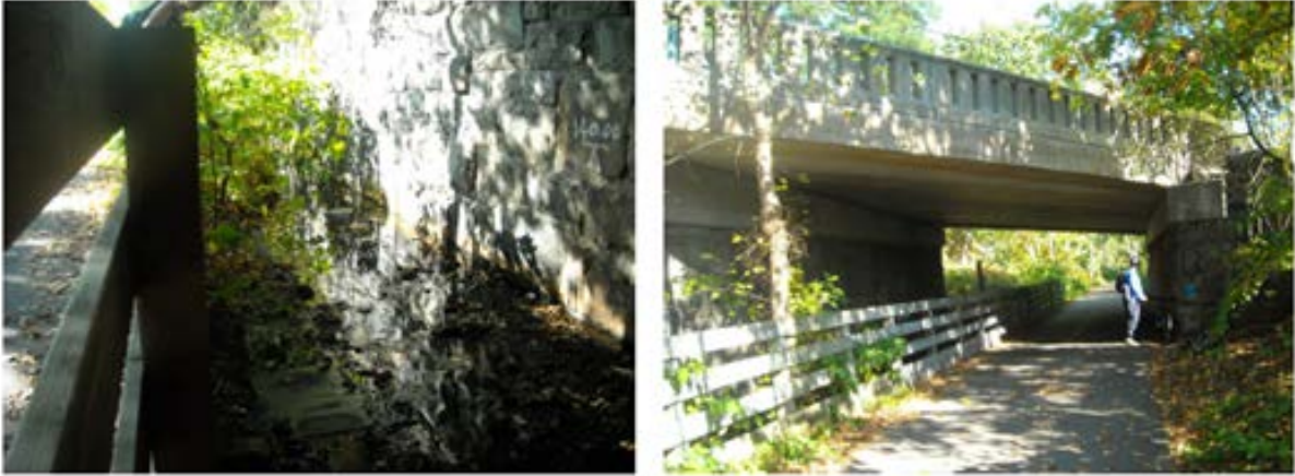
Figure 67. Existing images of Lowell Street Underpass
