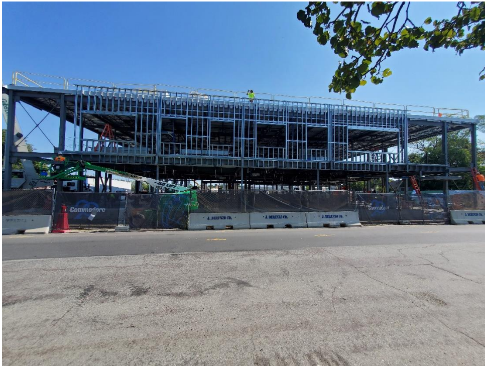
Photo # 5 – North Exterior Elevation at Building E (9/9/2022)
