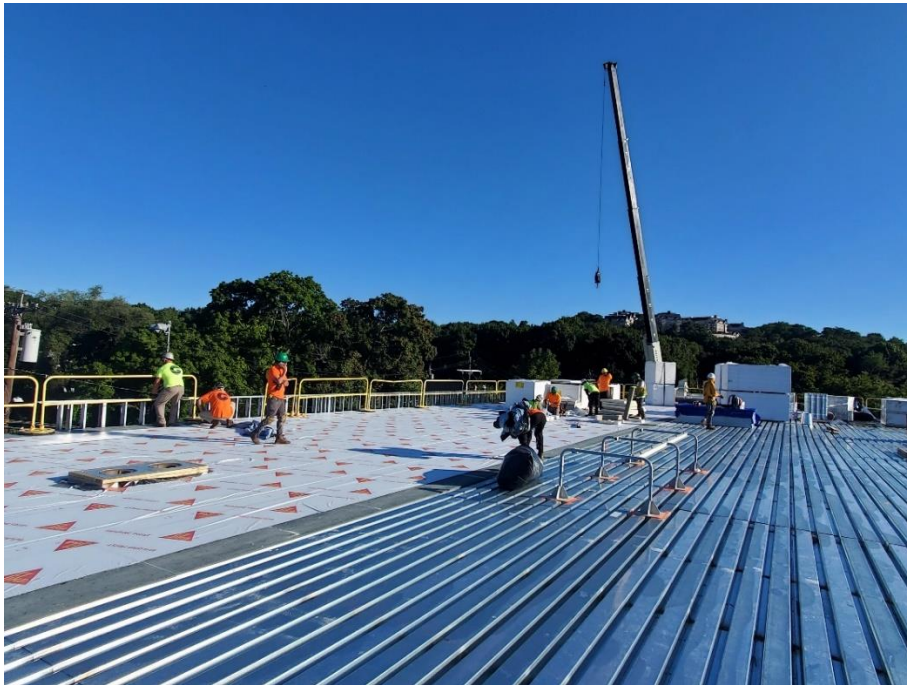
Photo # 3 – Membrane Roof System Installation (Roof Deck/Protection Board/AVB) at Building E (9/8/2022)
