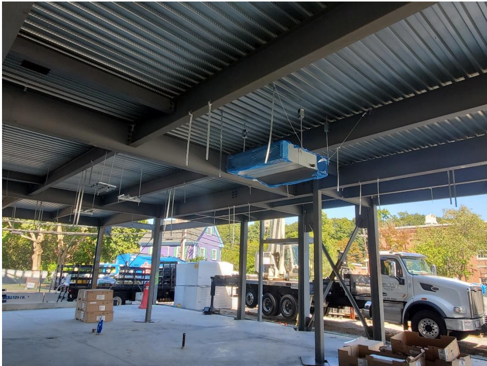
Photo # 1 – HVAC Rough-In at Building E (9/8/2022)
