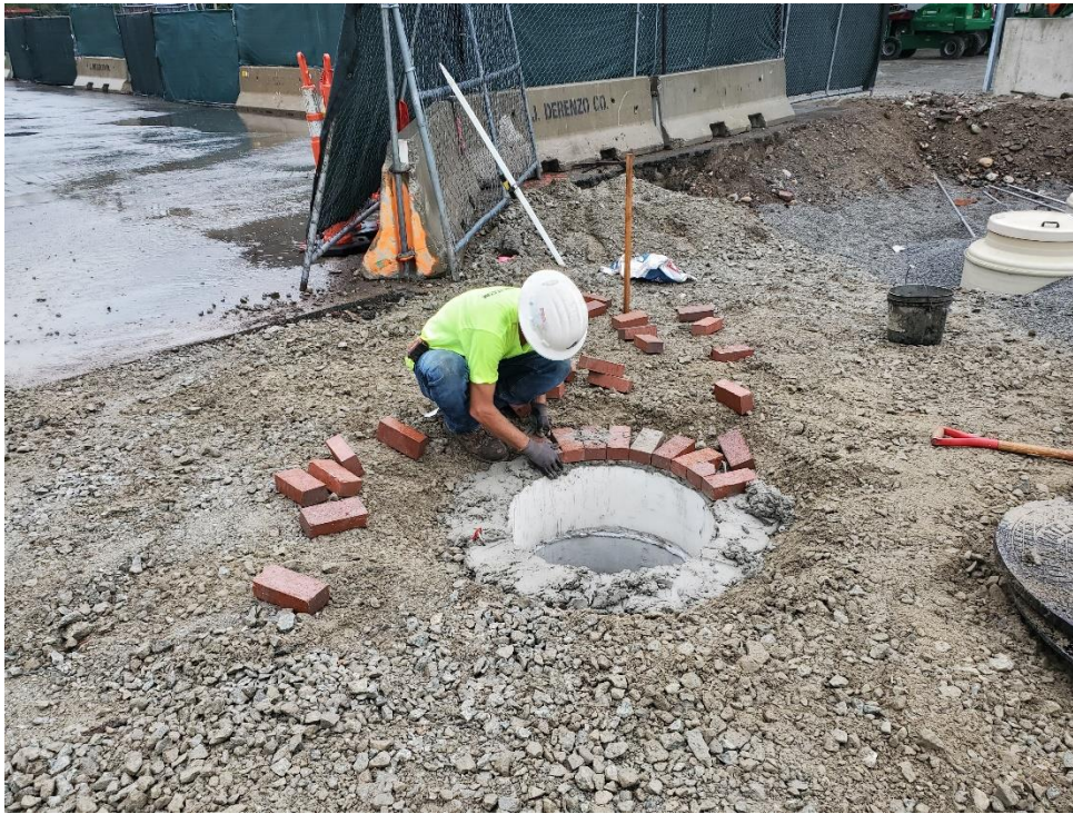
Photo #7 – Drainage Structure (9/13/22)
