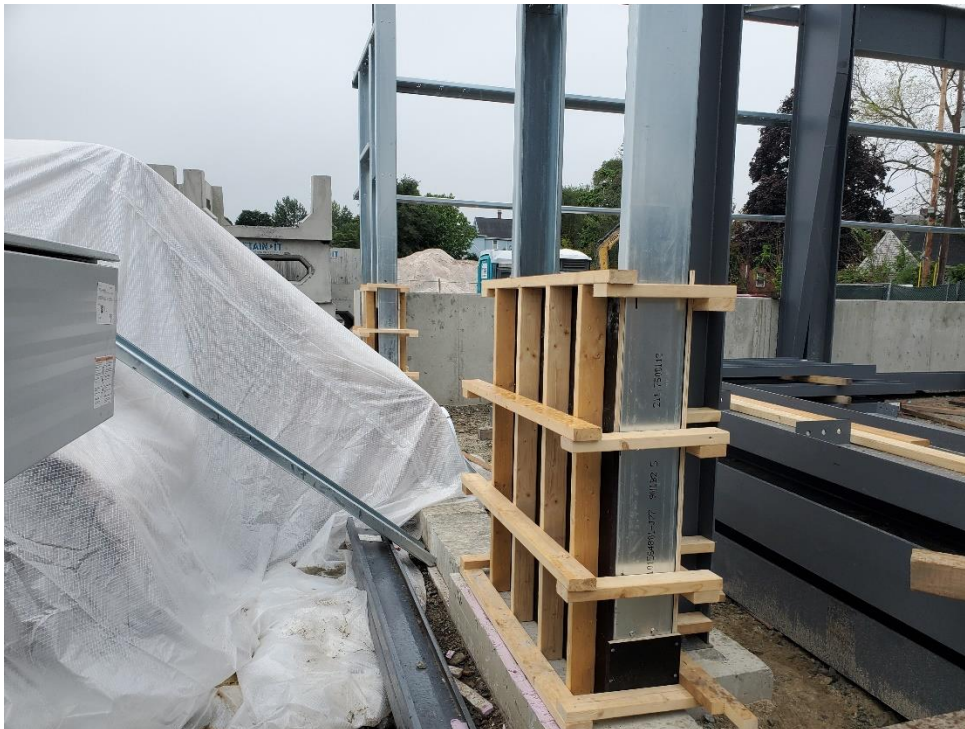
Photo #8 – PEMB Framing at Overhead Doors at Motor Equip. Repair Bays (9/13/22)
