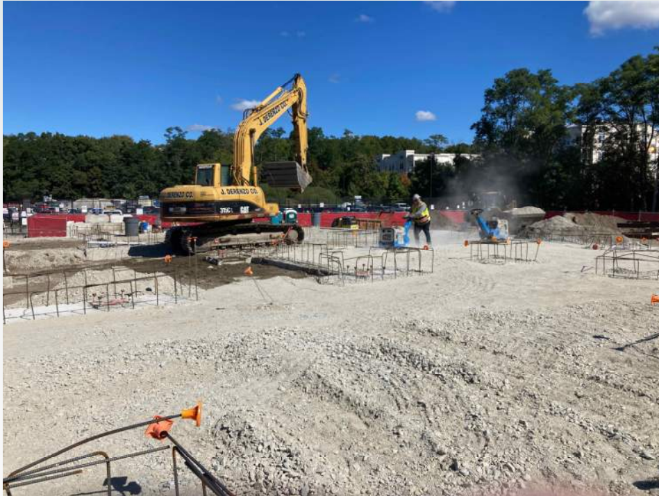
Bldg. C Backfill & Compaction
