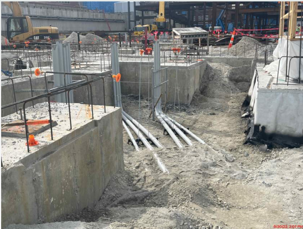
Underground Electrical & Plumbing
