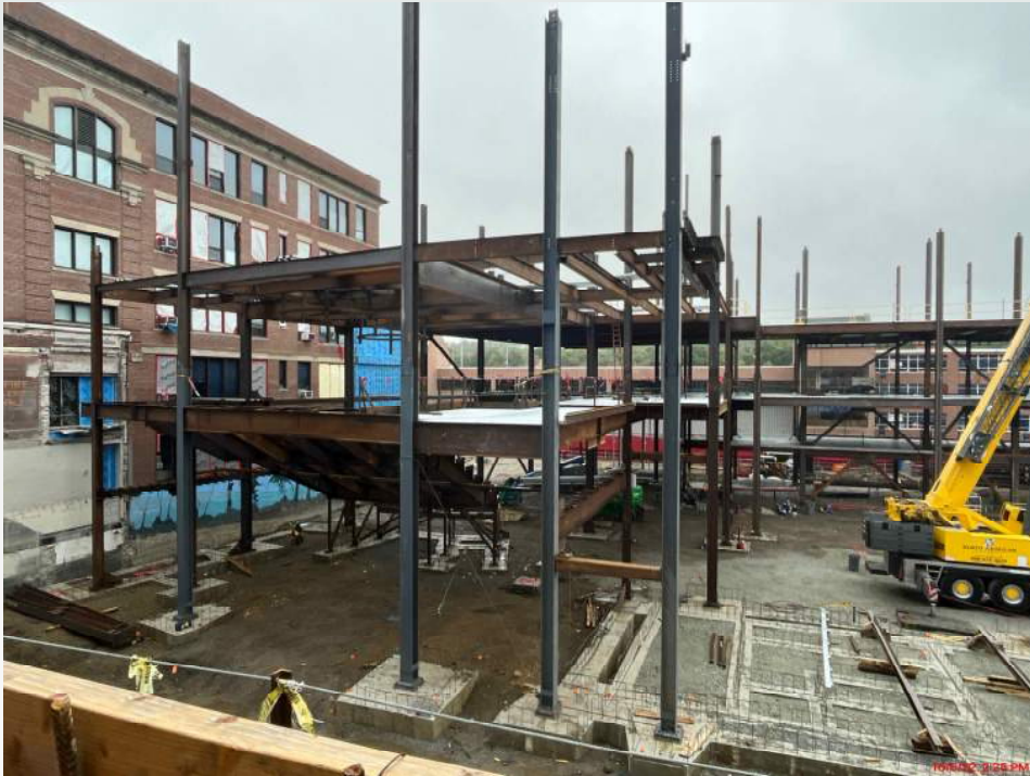
Building B Steel Erection
