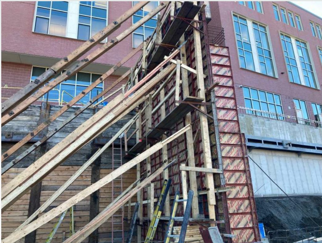
East High Wall Formwork
