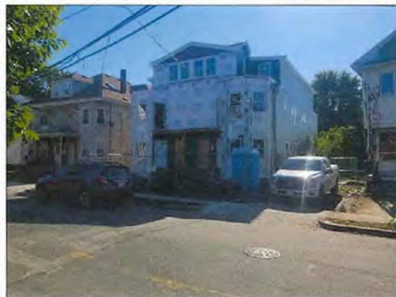
STREET VIEW OF 18-20 BELKNAP STREET
