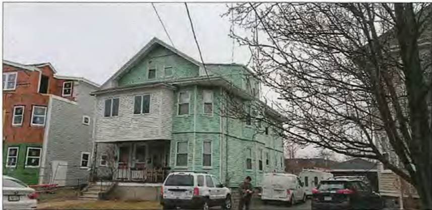
STREET VIEW OF 22-24 BELKNAP STREET
