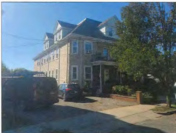
STREET VIEW OF 28-30 BELKNAP STREET
