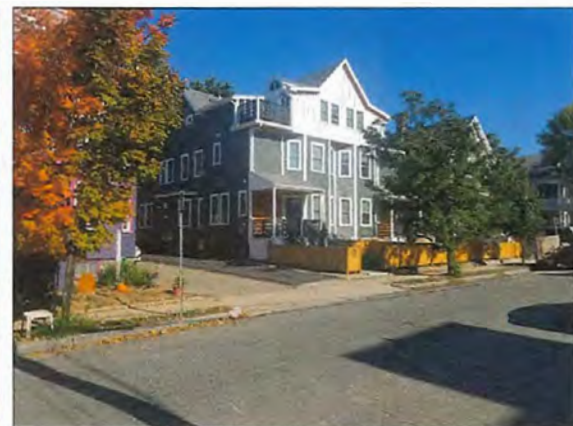
STREET VIEW OF 13-15 BELKNAP STREET
