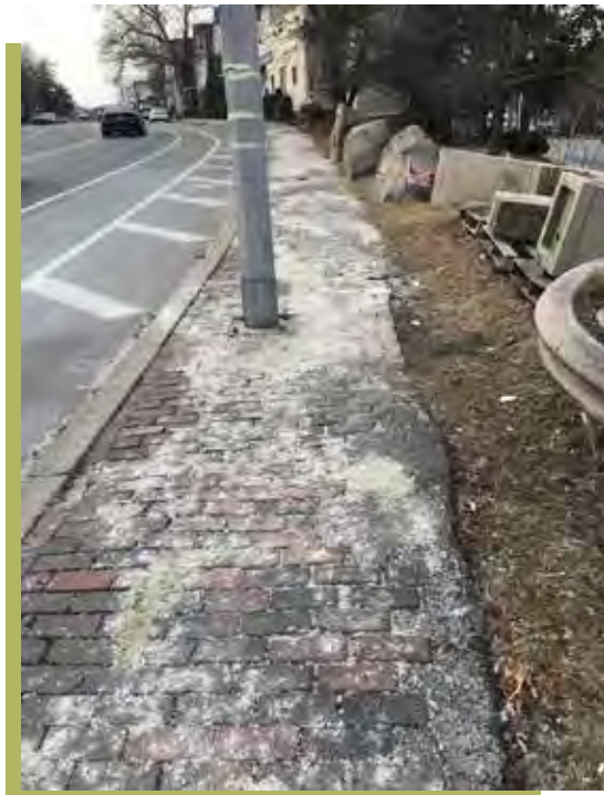
Figure 2 —Existing condition at Massachusetts Ave. looking west, January 2022
