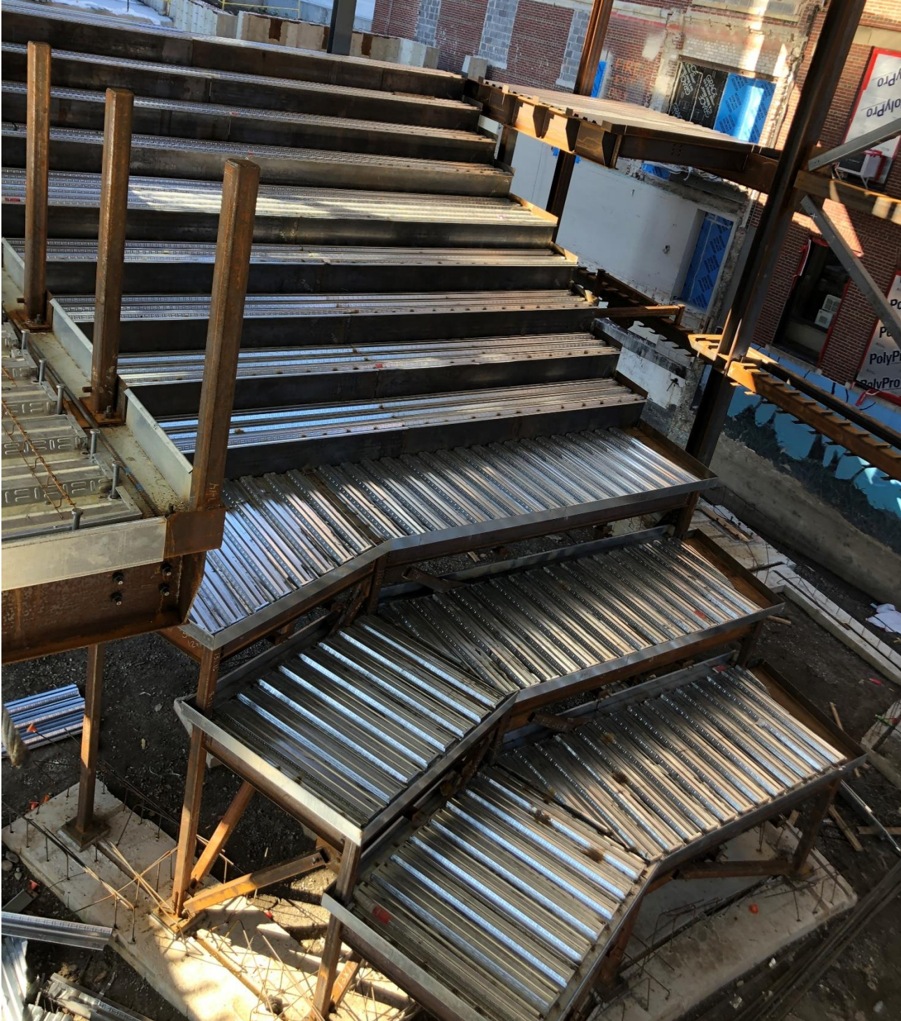
Photo 3: Forum Stairs Steel
