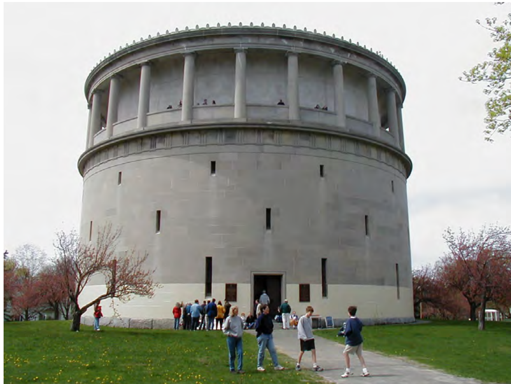
Park Circle Water Tower
