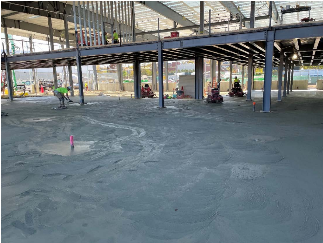
Photo #8 – Building E Maintenance Partial Slab on Grade (11/7/22)
