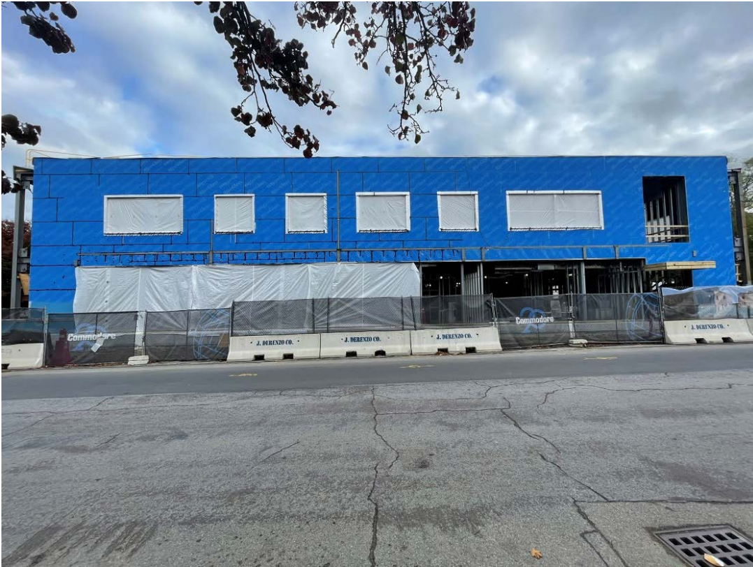
Photo #1 – Building E Admin. Front/Grove St. Elevation (11/1/22)
