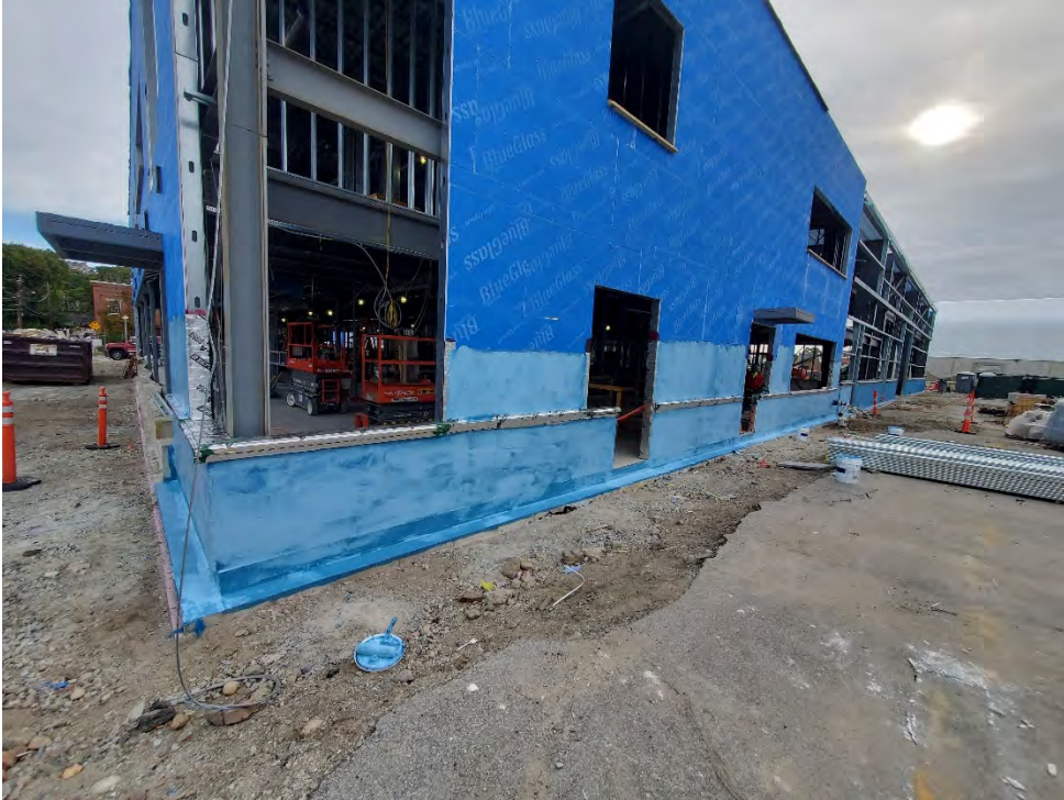
Photo # 1 – Building E: Water/Vapor Barrier (10/3/2022)
