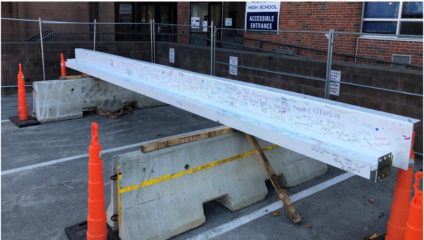
Photo 4: Topping off steel signed by the Senior Class
