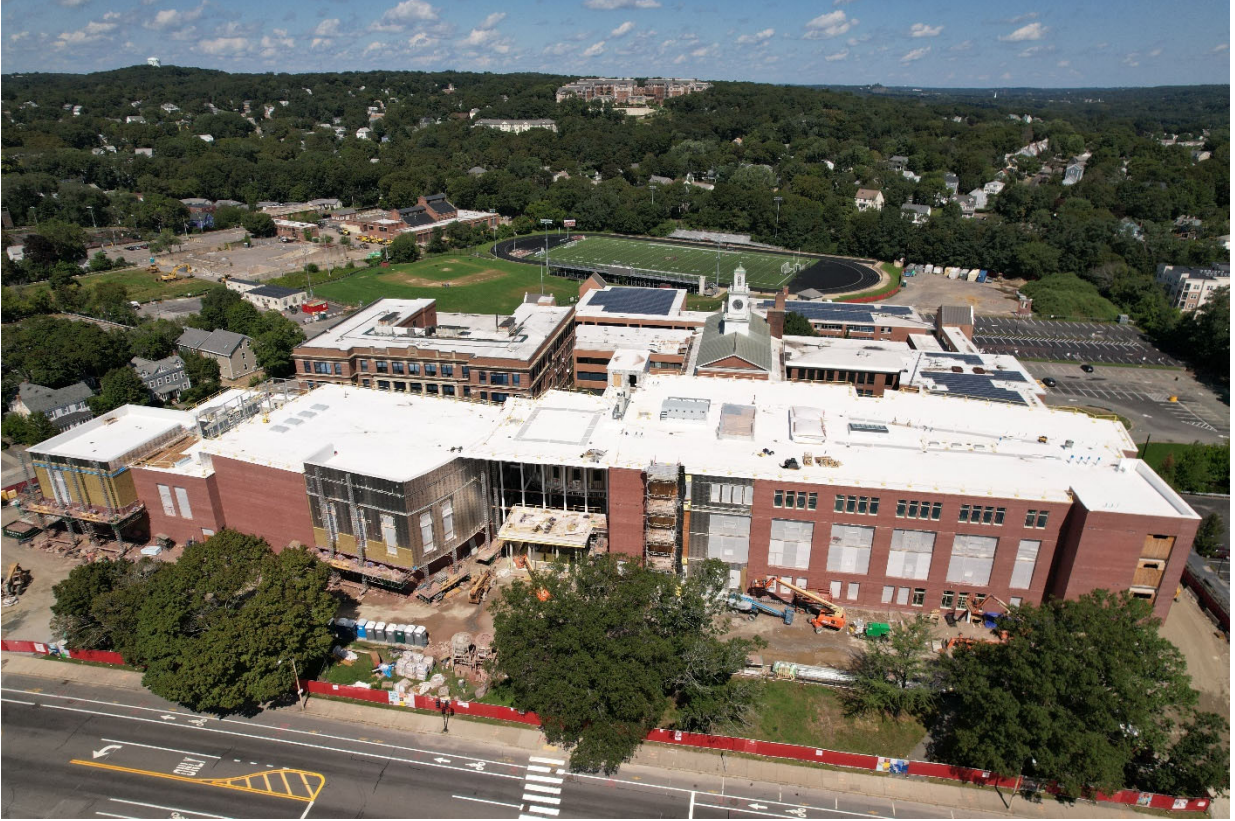
Arlington High School Building Project in progress
