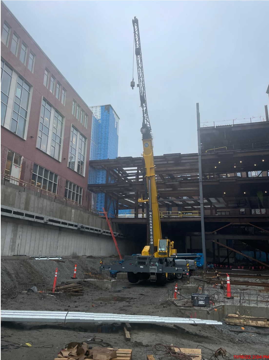
Photo 3: Steel connecting Phase 2 Building to Phase 1 Building
