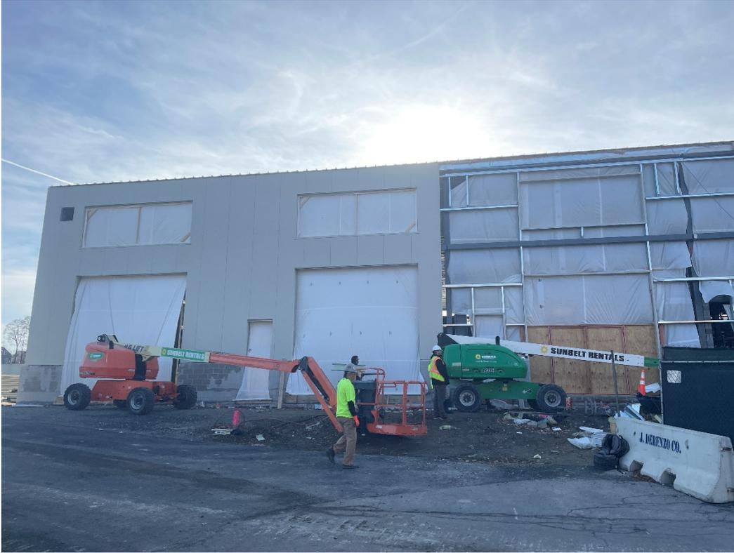
Photo #1 – Bldg. E Maintenance – Metal Siding Install (12/5/22)
