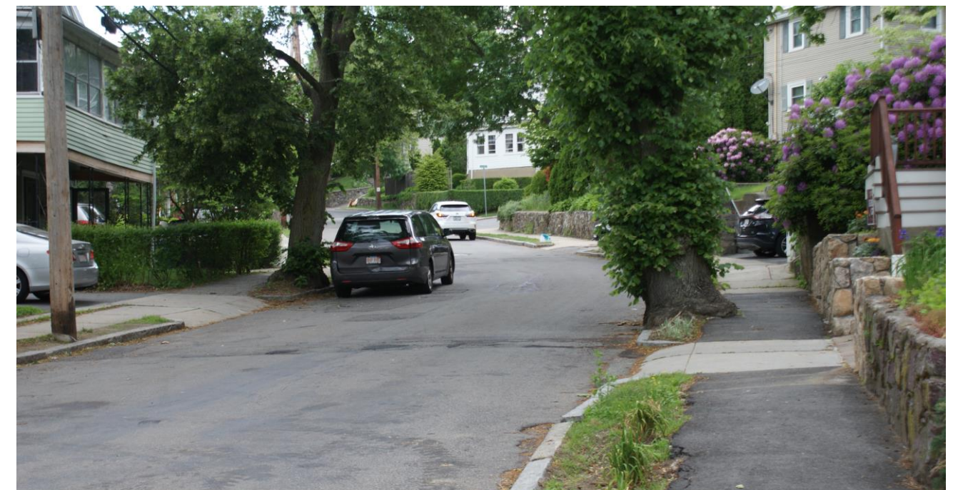
Horizontal/vertical alignment and on-street parking limit visibility.
