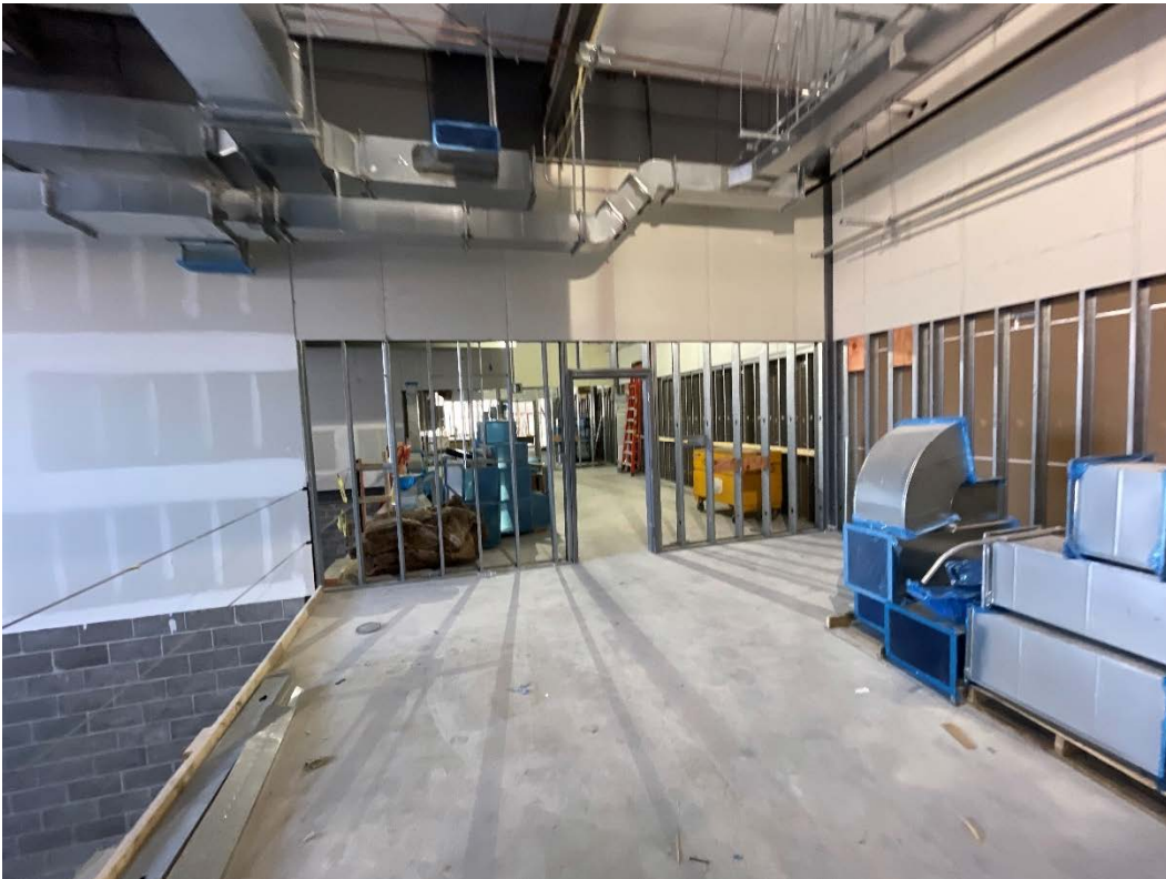
Photo #5 – Bldg. E Maintenance Mezzanine (1/9/23)
