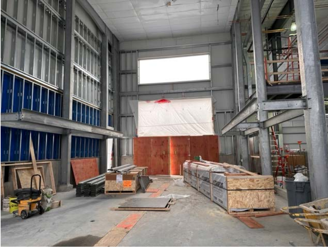
Photo #3 – Bldg. E Maintenance: Maintenance Bay (1/9/23)
