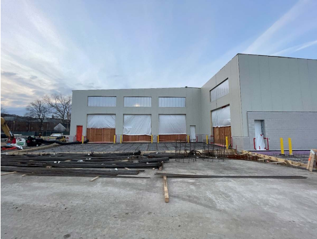
Photo #7 – Bldg. E Maintenance: Exterior Concrete Pour/SOG Apron (1/9/23)
