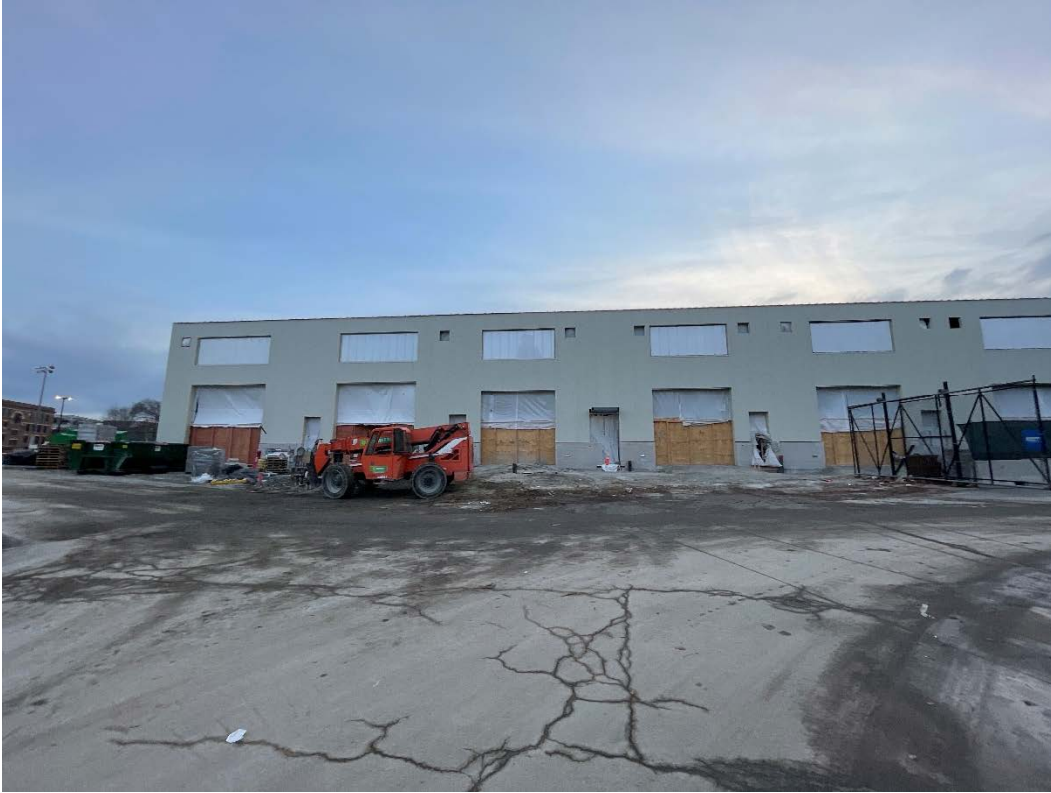
Photo #1 – Bldg. E Maintenance – Metal Panel Siding Installed (1/11/23)
