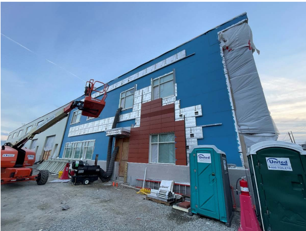
Photo #8 – Bldg. E Admin. – Exterior Terracotta Panel Install (1/11/23)
