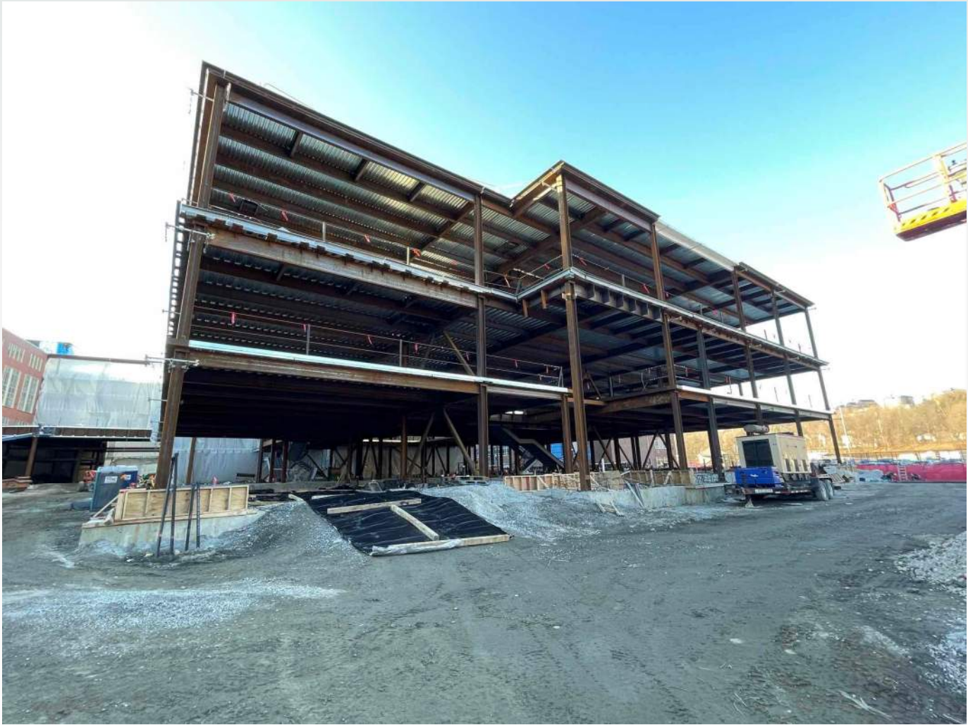
Bldg. C Steel Erection
