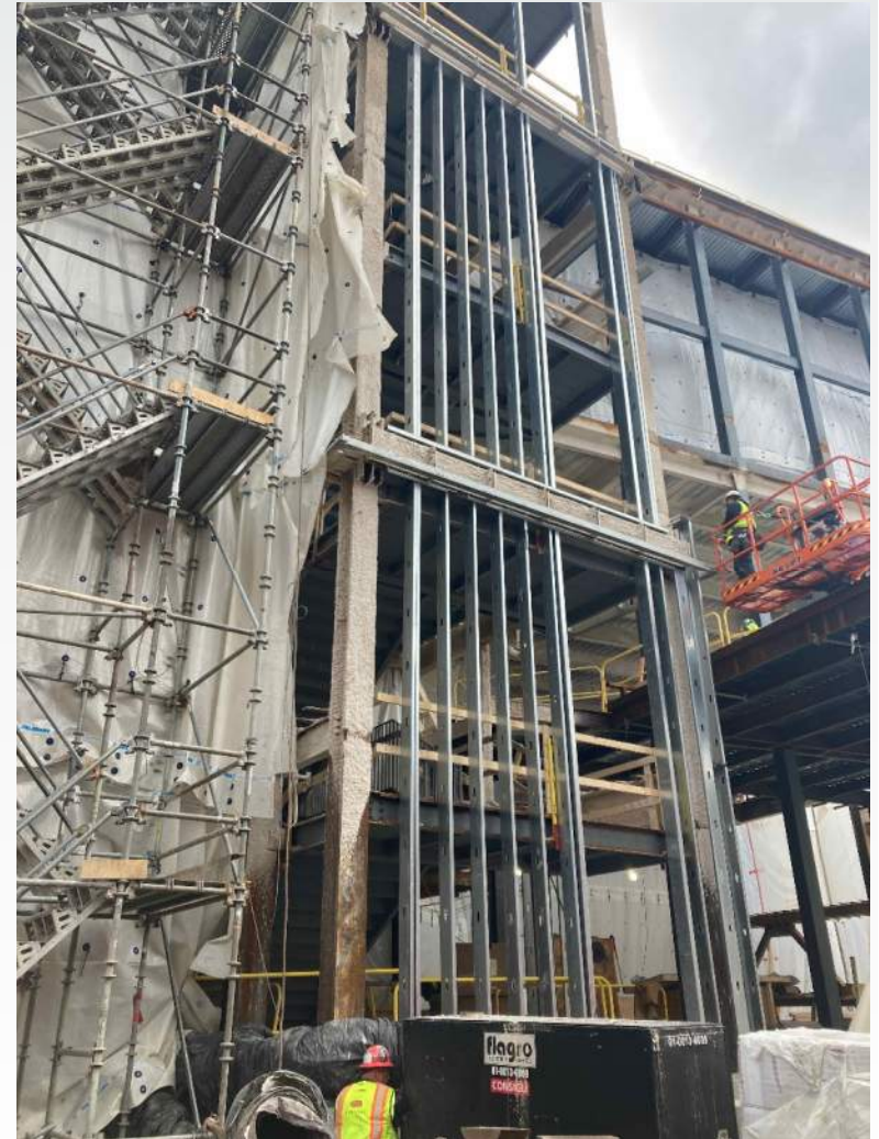
Exterior Framing Stair 1
