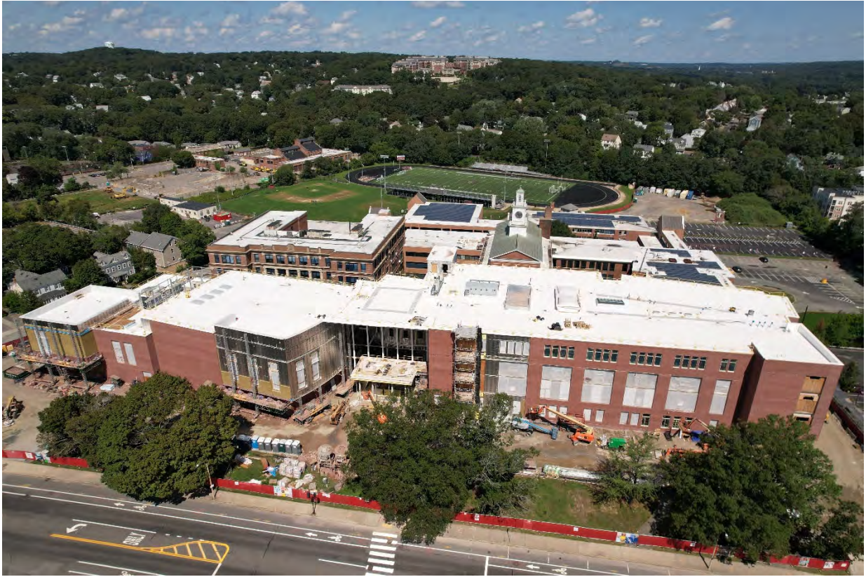
Arlington High School Building Project in progress
