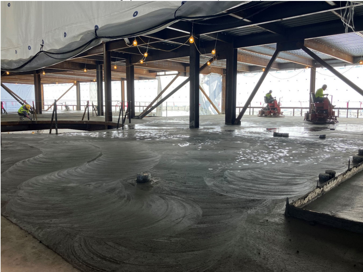
Photograph 2: Concrete Placement in Progress
