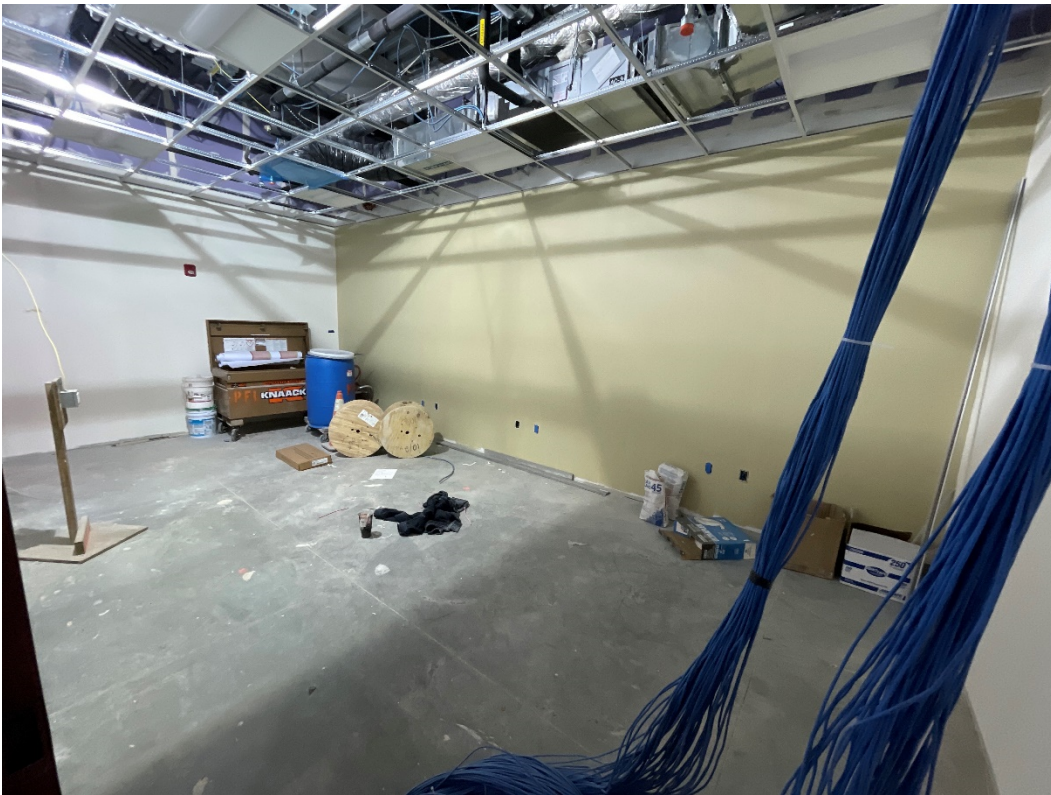
Photo #2 – Building E Admin. Finishes (2/6/23)
