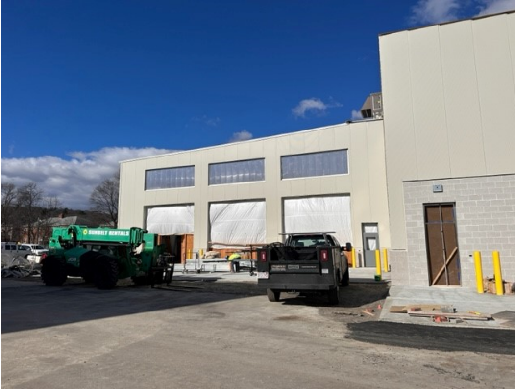
Photo #7 – Bldg. E Maintenance Washbay from South Elevations (2/14/23)
