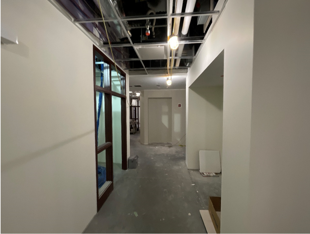
Photo #1 – Building E Admin. Finishes (2/6/23)
