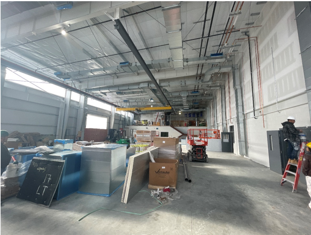
Photo #4 – Building E Maintenance General Workshop (2/6/23)
