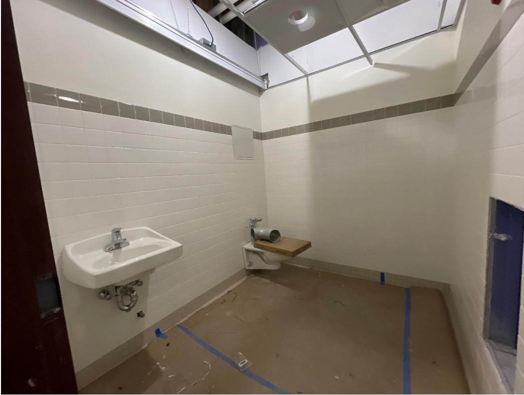
Photo #3 – Building E Admin. Bathroom Finishes (2/6/23)
