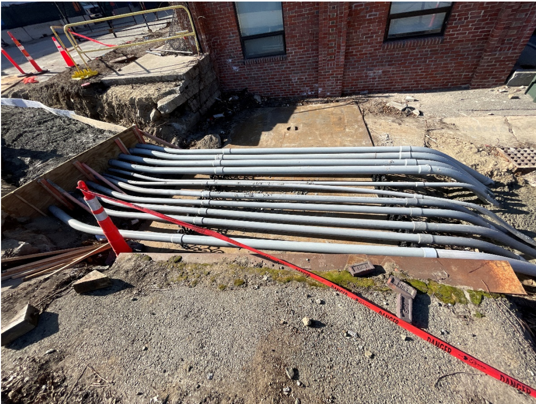
Photo #8 – Primary Electrical Conduits & Teldata (2/14/23)
