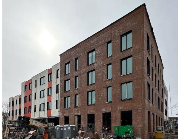
1005 Broadway Chelsea, MA | 38 Units PHIUS Pre-certified, In Construction
