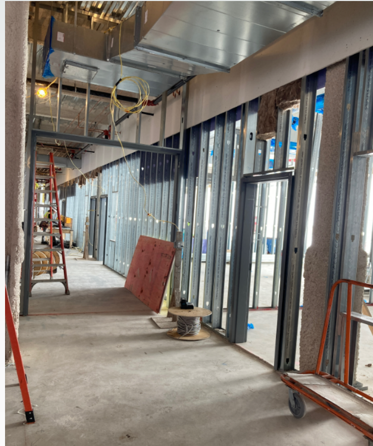
MEP Rough (BLDG B; Level 3)
