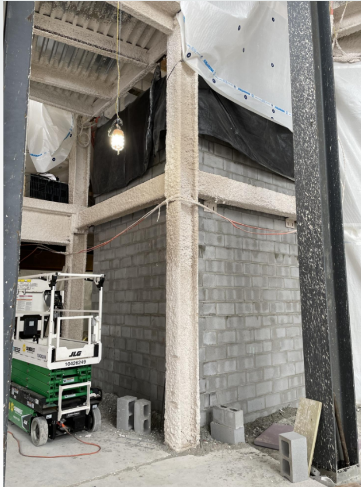
Elevator Shaft Install (BLDG B; Elevator 1)
