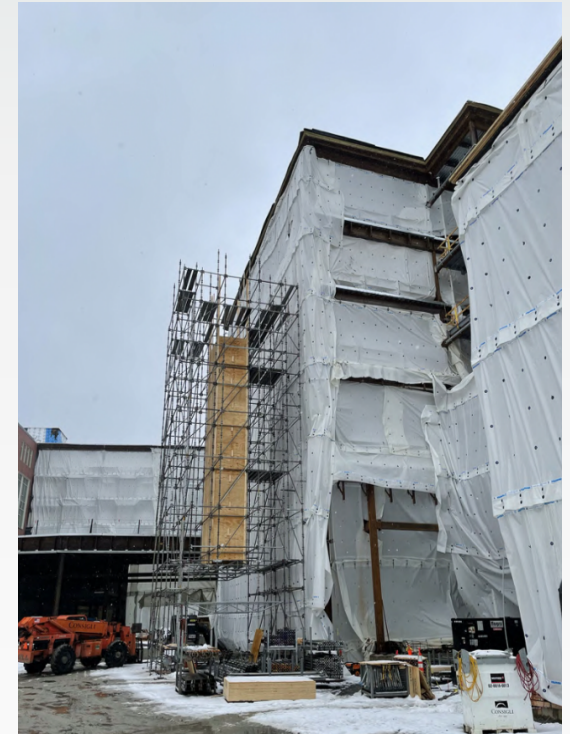
BLDG B (South Elevation) Tarpred
