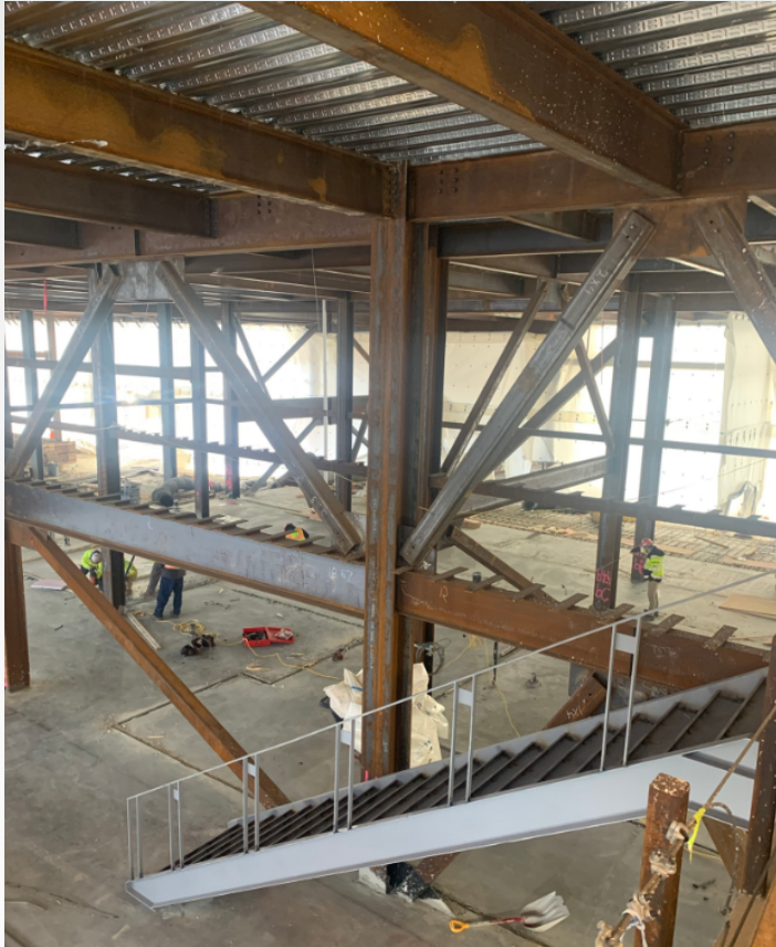
Slab on Grade Placement + Stair 12 Install
