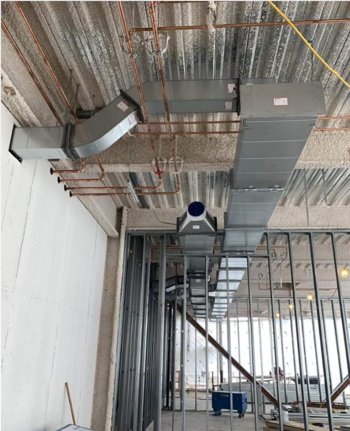
MEP Rough (BLDG B; Level 2)
