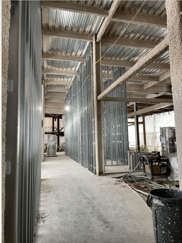
Interior Framing (BLDG B; Level 1)
