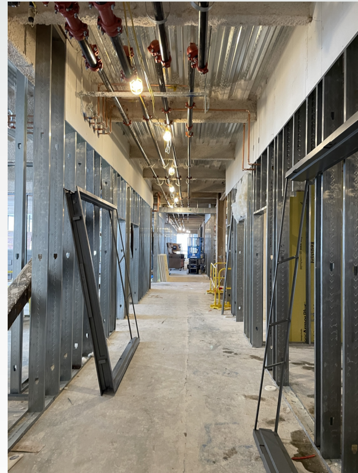
Interior Framing (BLDG B; Level 3)
