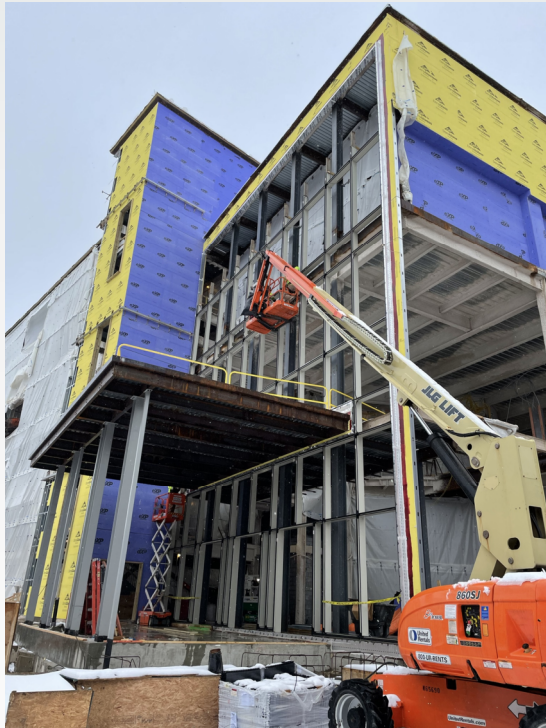
Exterior Sheathing + Curtainwall Frames (BLDG B; Main Entry)
