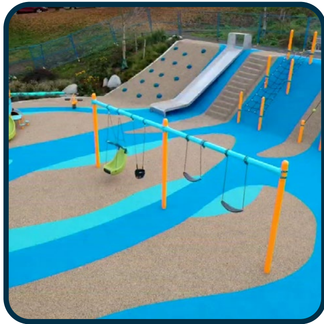
Poured-in-Place Rubber Safety Surfacing (as recommended by Comissioners and Volunteers of the Arlington Disability Commission)
