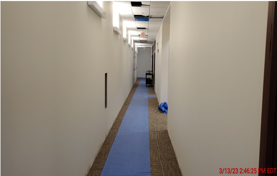
Photo #4 – Building A Finishes (3/13/23)
