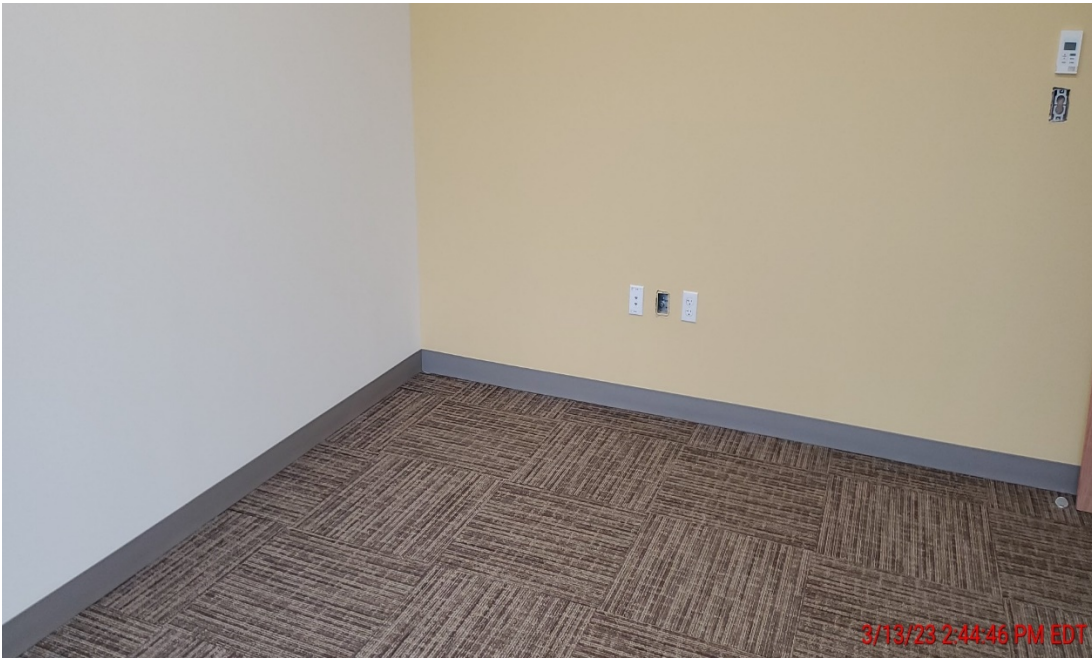
Photo #3 – Finishes: Carpet & Wall Base (3/13/23)
