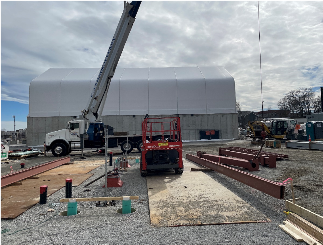
Photo #7 – Fuel Island Canopy Erection (3/7/23)
