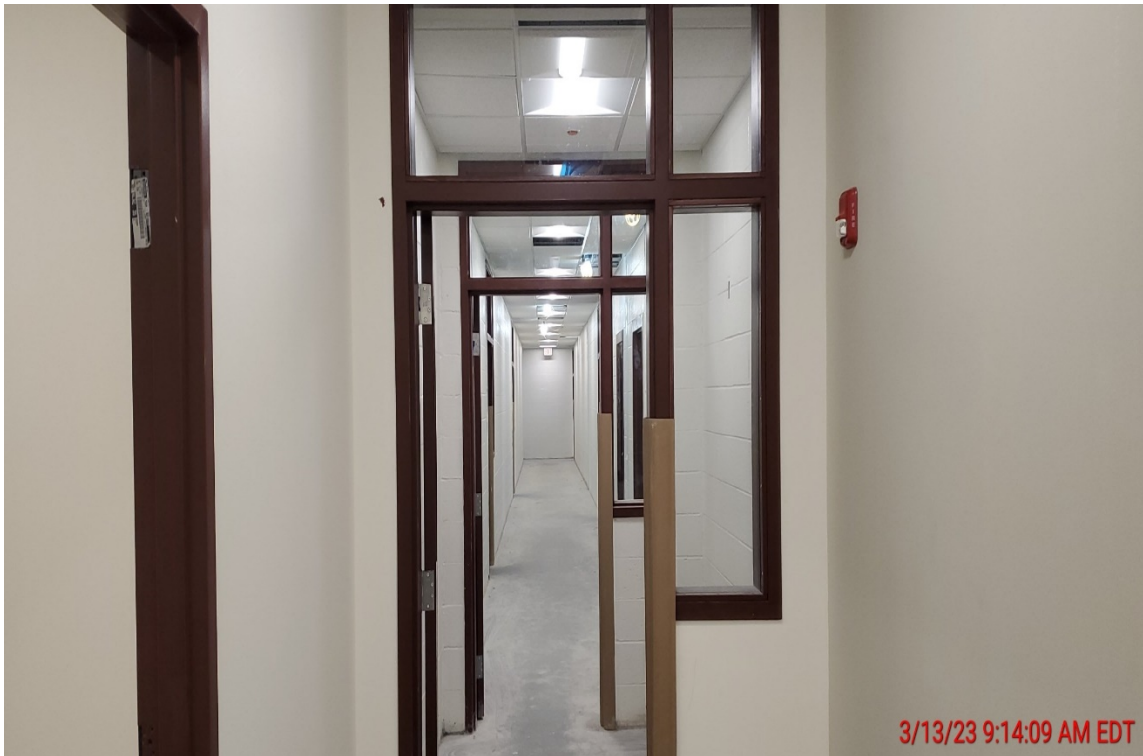
Photo #6 – Building A Corridor (3/13/23)
