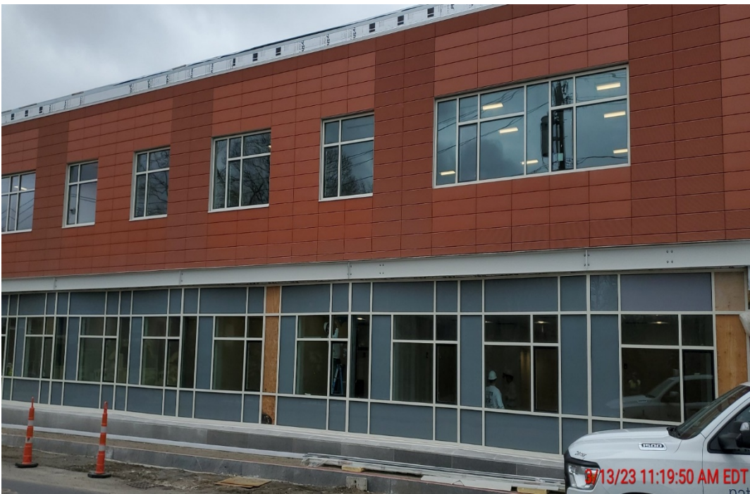
Photo #2 – Building E View from Grove Street (3/13/23)
