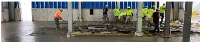
Building E pouring of concrete floor slab.
