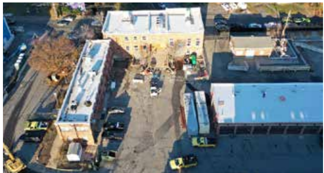
Site overview – Bldg A (on Grove Street), Bldg B (left side), Bldg C (right side).
