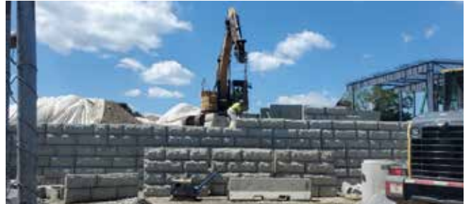
Construction of retaining wall.
