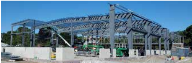
Building E steel erection.
