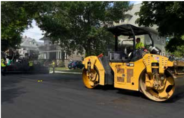
Pavement preservation on Medford Street, spring 2022.
