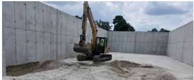
Preparation of Salt Shed floor.
