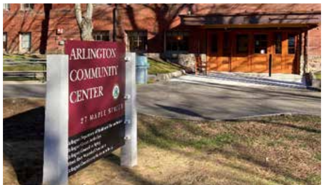
Maple Street main entrance – new sign, entry, canopy.
