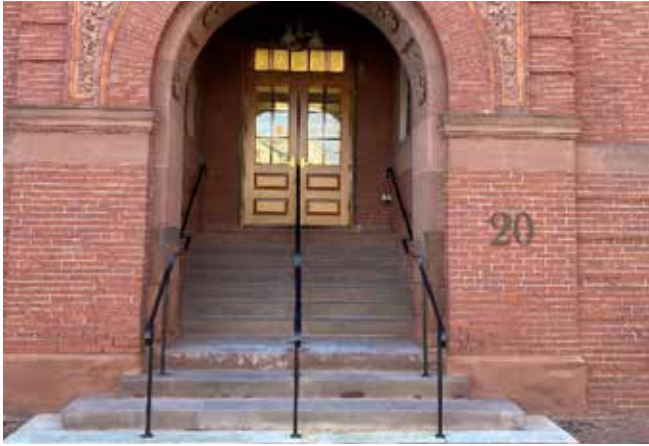
Academy Street entrance – new stairs, doorway.
