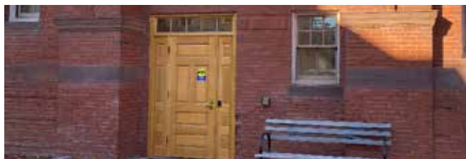
New East entry with accessible door controls.
