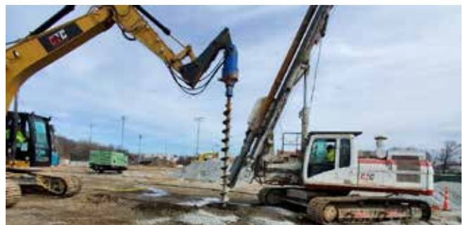
Site work – drilling exploratory holes.
