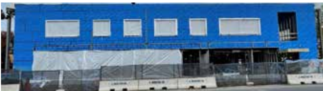
Building E exterior from Grove Street – finished exterior will be terracotta tile.
