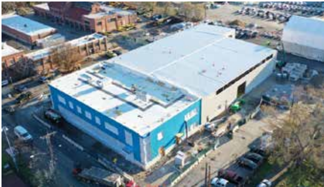
Site overview – new Building E in late 2022.
