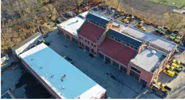
Site overview – Building D.
