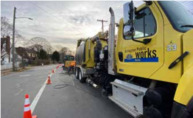
Water Division on site fixing a water main break.
