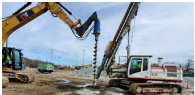
Site work – drilling exploratory holes.
