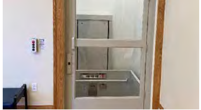
New accessible lift connecting East entry with ground and first floors.
