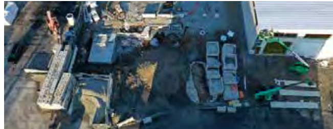
Discovery of large retaining tank adjacent to Building E.
