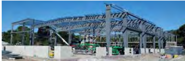
Building E steel erection.
