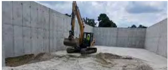
Preparation of Salt Shed floor.
