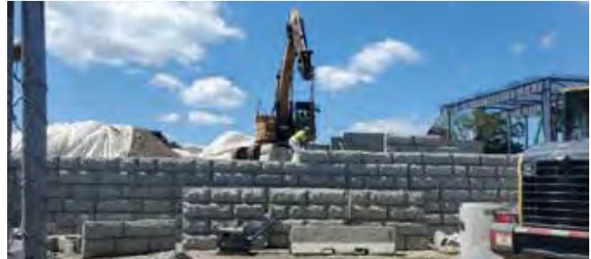
Construction of retaining wall.
