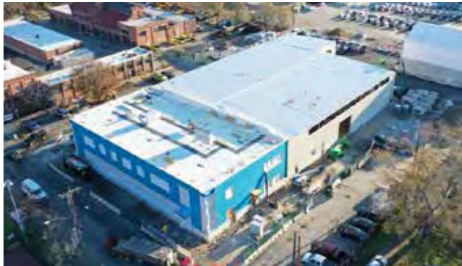
Site overview – new Building E in late 2022.
