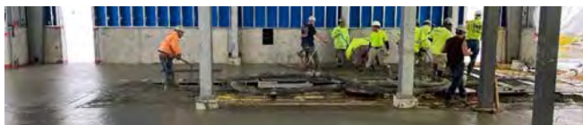
Building E pouring of concrete floor slab.
