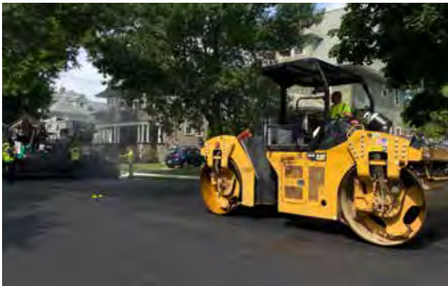
Pavement preservation on Medford Street, spring 2022.
