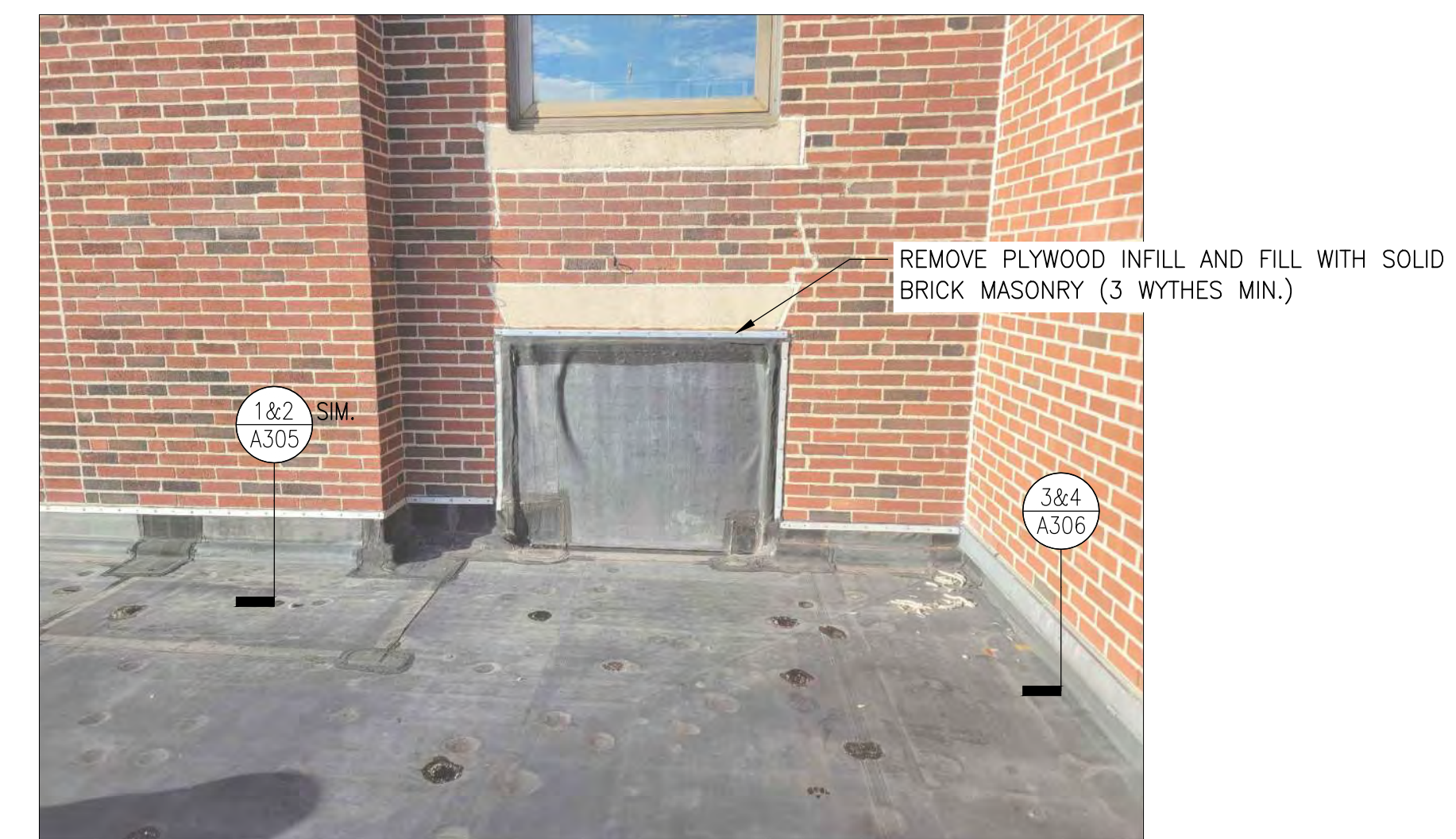
2 ABANDONED WINDOW DETAIL ROOF D
