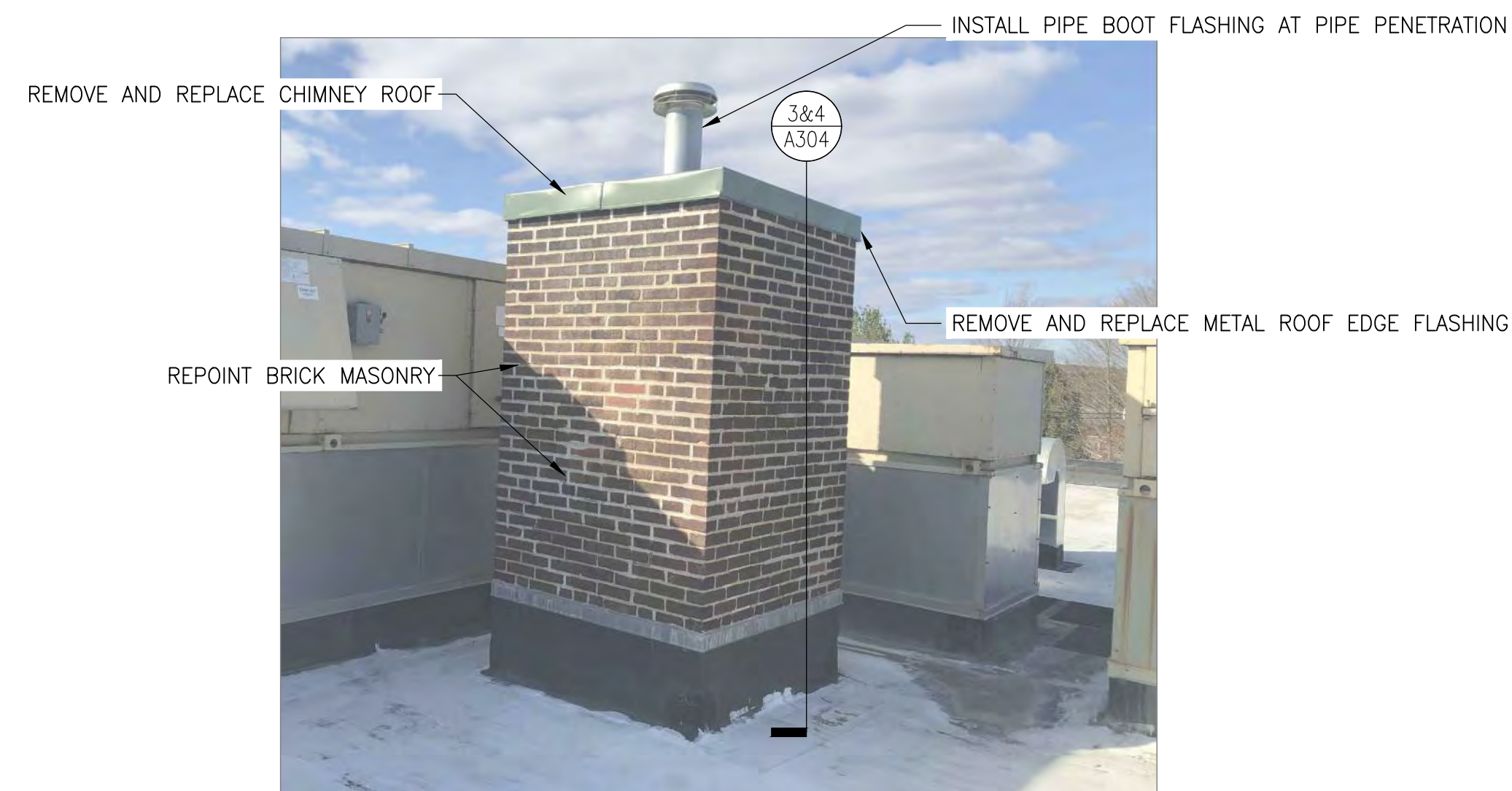
1 BRICK CHIMNEY DETAIL ROOF A
